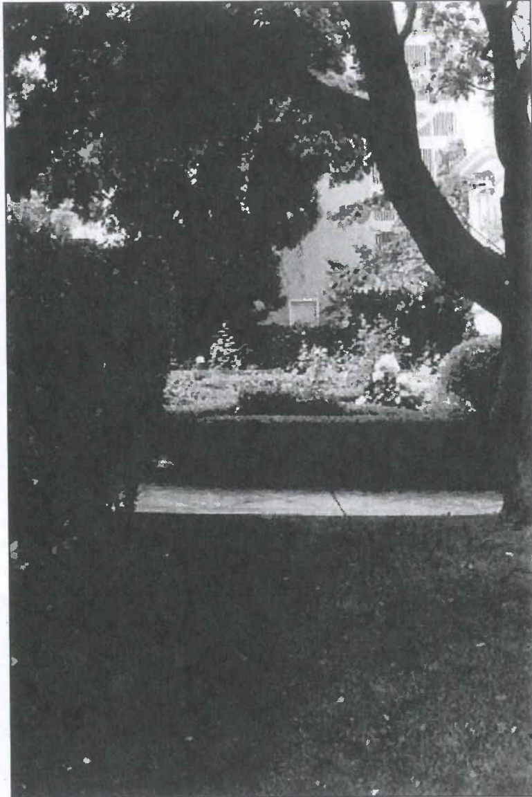
Photo 9. Burr House, 1772 Vallejo Street, 94123. Site, view west. Note area with box hedges, site of unreinforced masonry retaining wall.
