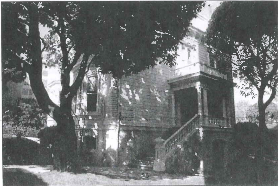
Photo 7. Burr House, 1772 Vallejo Street, 94123. Site, view northwest. Note mature trees planted adjacent to porch foundation and tree limbs encroaching on house
