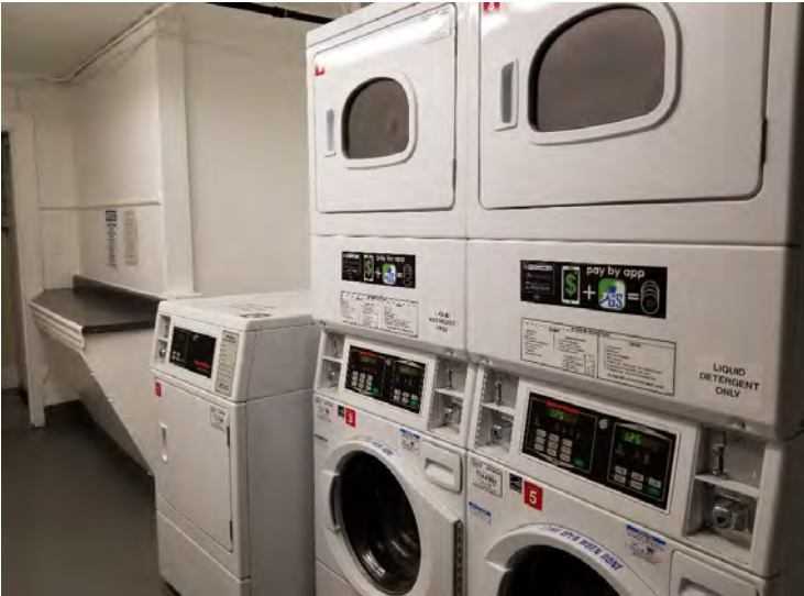
Photo: Union laundry room
