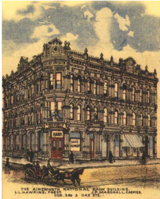
Ainsworth Building, Portland, Oregon 1881. Source: pcad.lib.washington.edu/building/15374/
