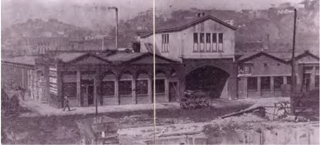
Davis Street façade circa 1910s. The six bays on the left of the central arch (2 rectangular and 4 arched) as well as the center arch appear to be original. The openings to the right of the center arch are post-1906 construction. The second story was destroyed in the fire and not replaced. Author's collection.
