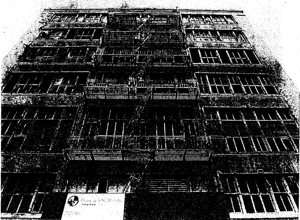
View of Stevenson Street façade looking up
