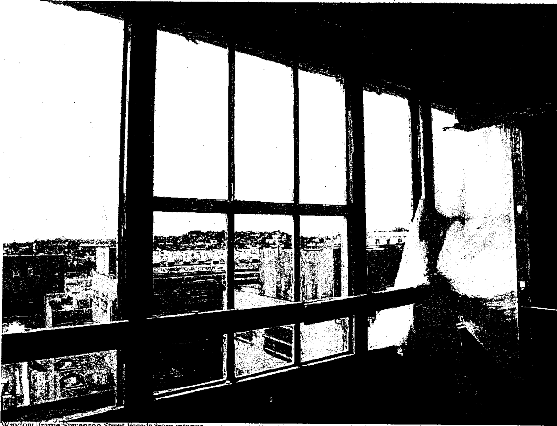
Window Frame Stevenson Street Facade from interior
