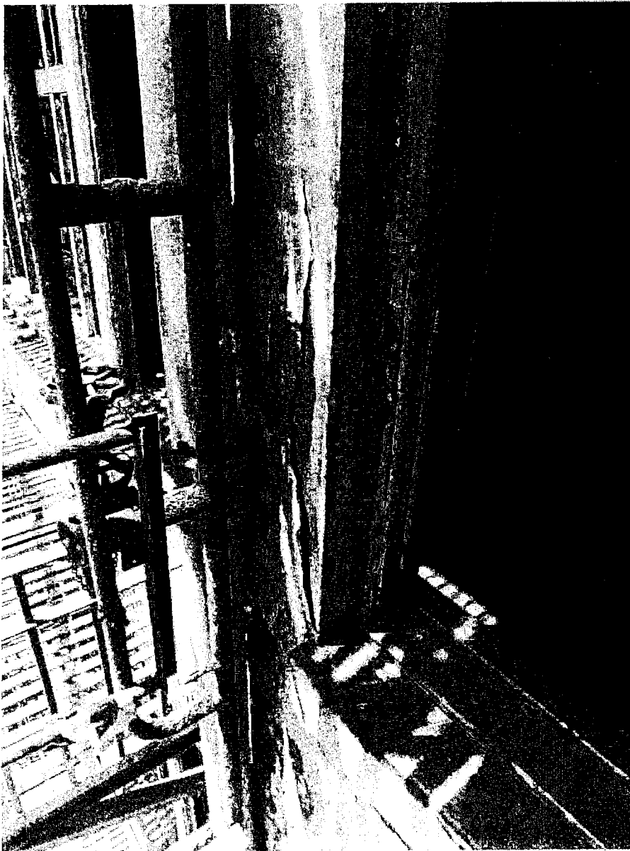
Typical spalling at parged concrete
