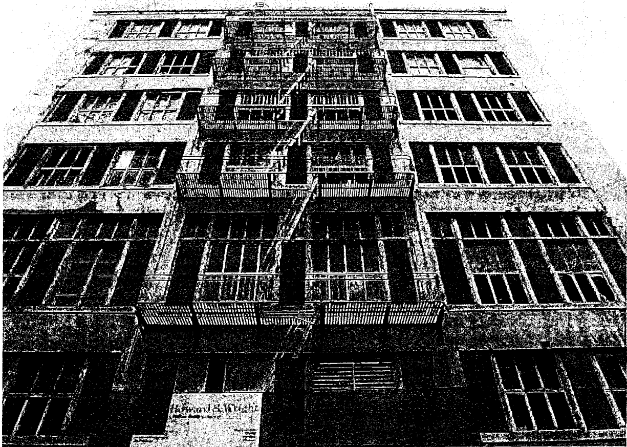
View of Stevenson Street façade looking up showing typical locations of double hung sash being replaced with new wood double hung sash. (Replaced sash areas shown in RED).
