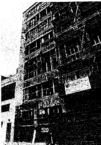
Stevenson Street Facade (Southwest Corner)
