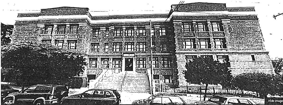
Figure 70. Former Lowell High School (now San Francisco City College’s John Adams Campus).
