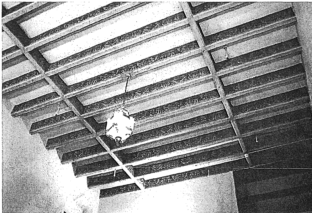
Figure 35. Ceiling of main lobby/stair; view toward north.
