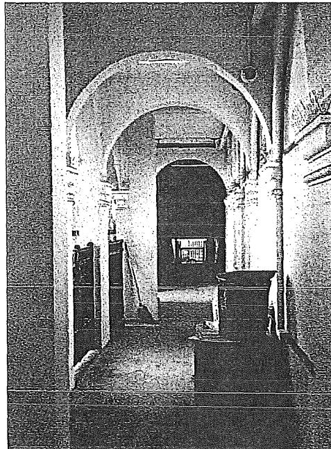
Figure 30. Passage at first floor level; view toward east.
