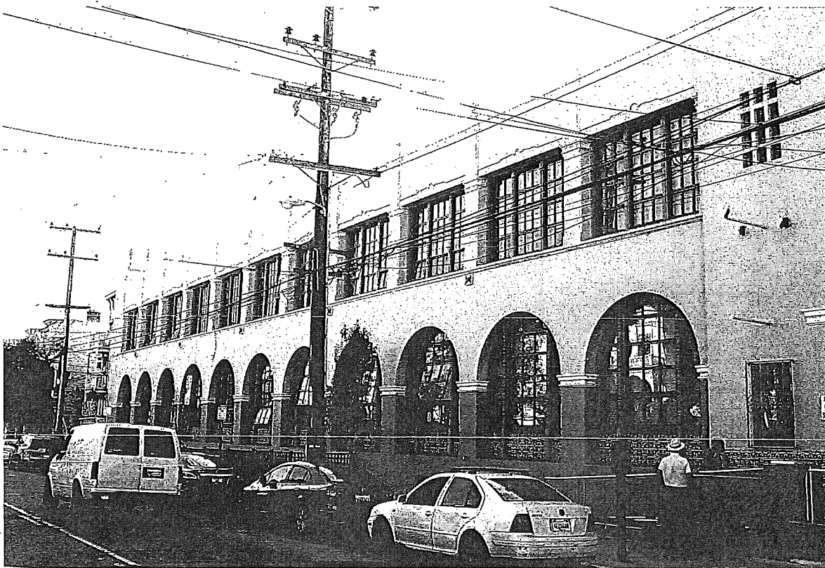
Figure 14. East façade of the Sunshine School (classroom wing); view toward southwest.
