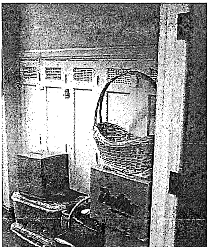
Figure 41. Original lockers in classroom.
