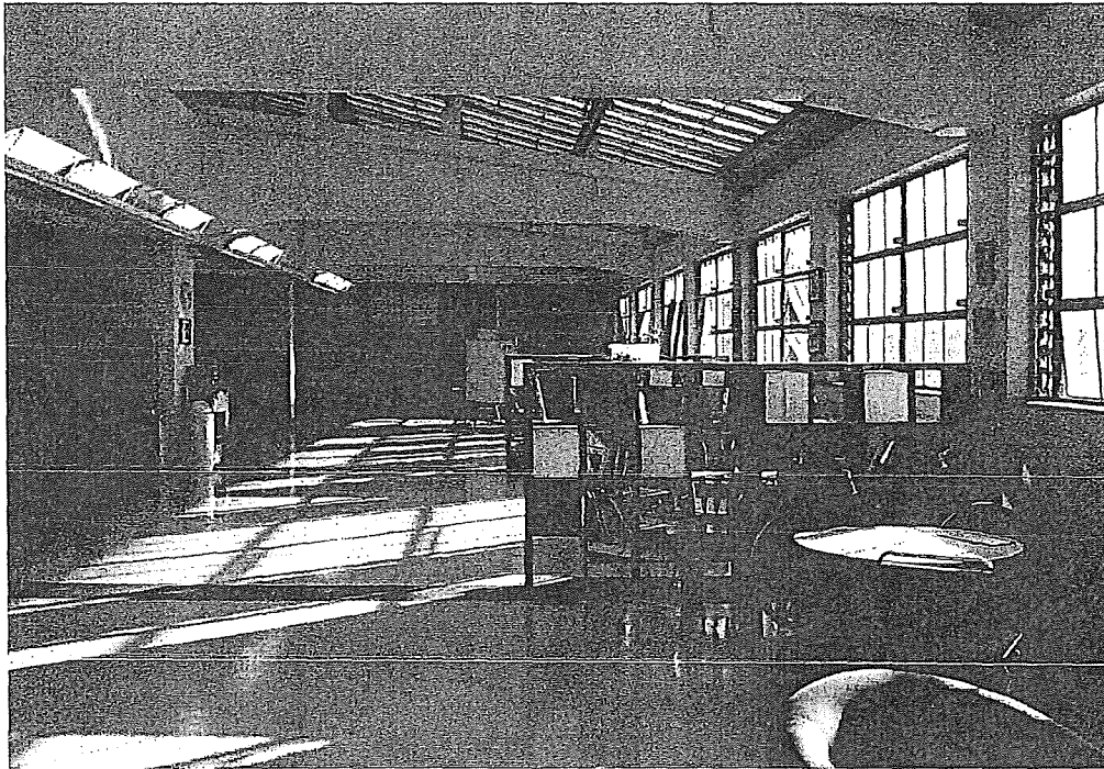
Figure 43. Typical corridor on second floor level; view toward south.
