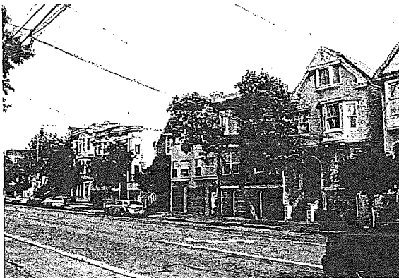
Figure 4. The east side of Bryant Street across the street from the former Sunshine School; view toward northeast.
