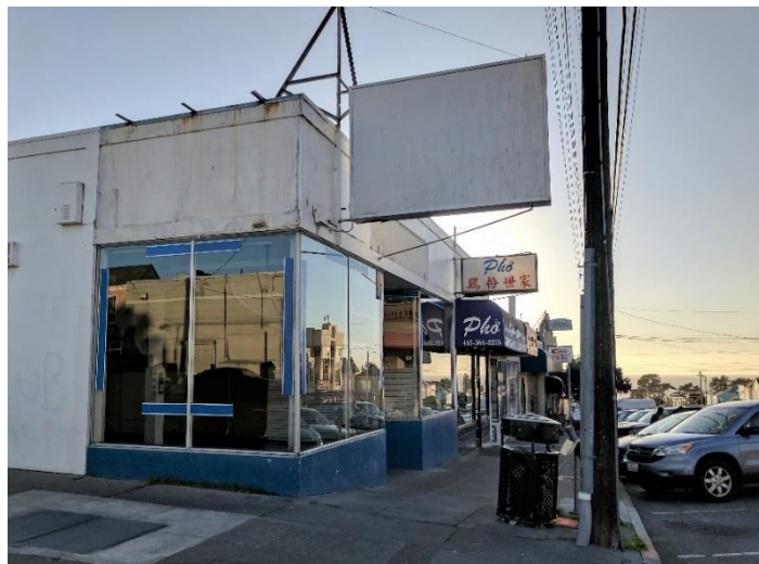
Inset Figure 1. Existing Storefront at 2505 Noriega
