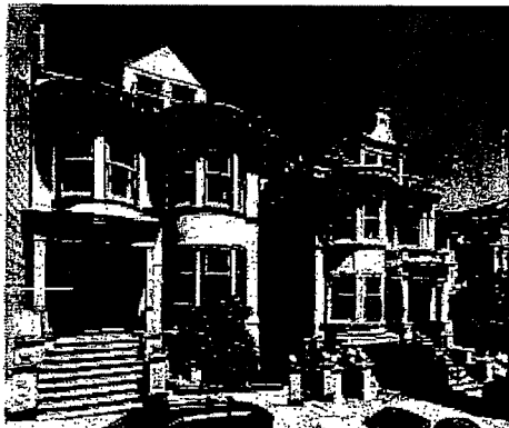
1080-1082 and 1086-1088 Fulton Street, designed by August Nordin and completed in 1902. (Google Maps)
