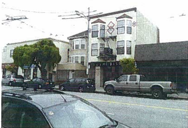
Subject property and buildings 100' to the East along Balboa Street
