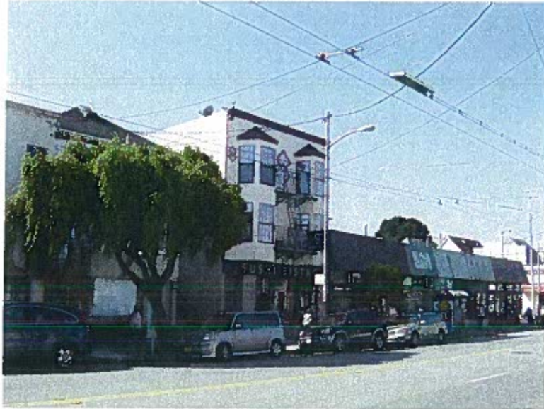
Subject property and buildings 100' to the West along Balboa Street
