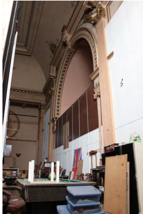
FIGURE 32. CHURCH: SANCTUARY SHOWING SEALED ALTAR NICHES, 2016.
