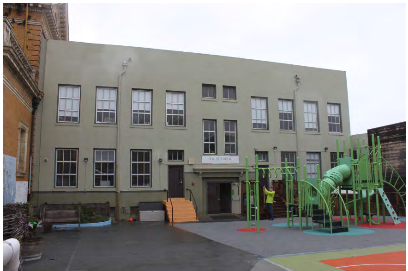
FIGURE 45. SCHOOL: REAR (SOUTH) ELEVATION AND SCHOOL YARD, 2016.
