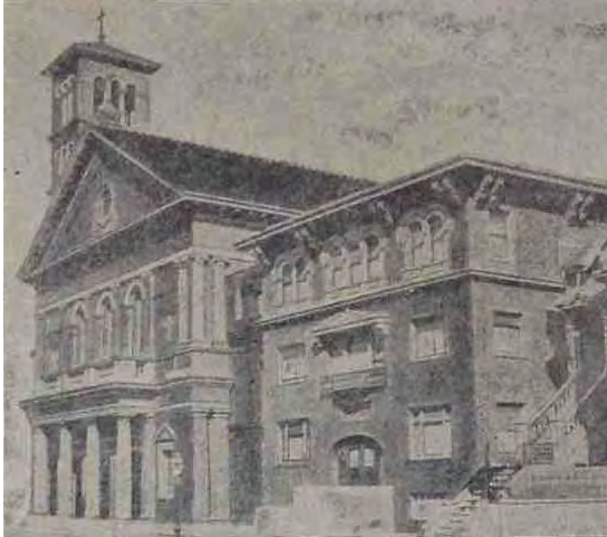
FIGURE 58. CHURCH AND RECTORY SHOWING ORIGINAL DOOR AND WINDOW TREATMENT ON FIRST AND SECOND STORIES. SOURCE: CATHOLIC MONITOR, OCTOBER 2, 1920
