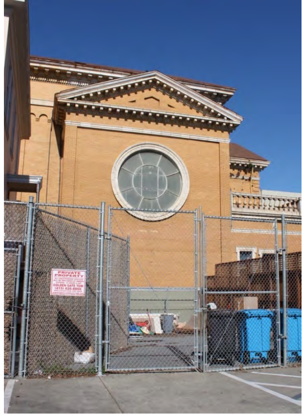
FIGURE 11. CHURCH: SOUTH TRANSEPT AND SACRISTY LOOKING NORTH FROM PARKING AREA OFF OAK ST., 2015.
