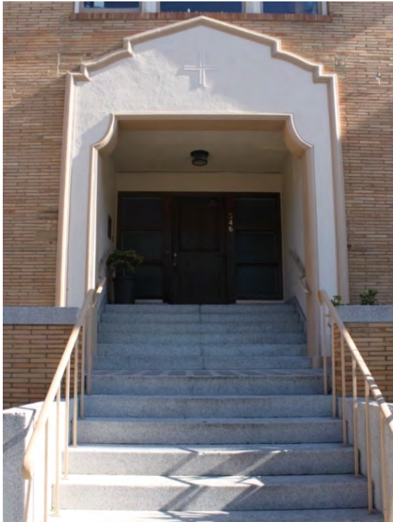
FIGURE 39 (LEFT). RECTORY: MAIN ENTRANCE, 2015.
