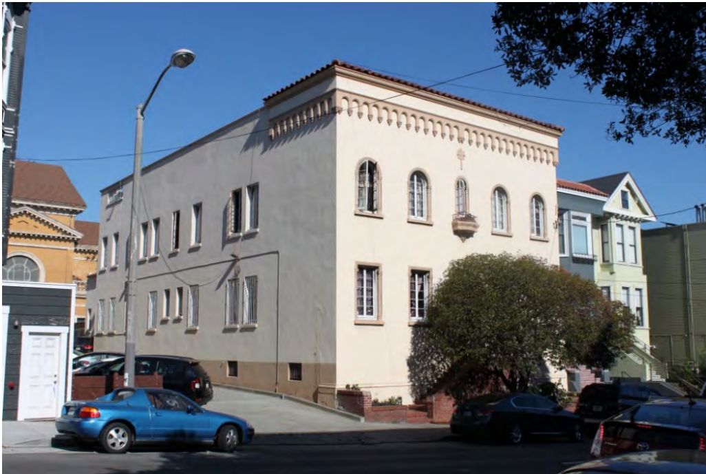
FIGURE 47. CONVENT LOOKING NORTHEAST FROM OAK ST., 2015.
