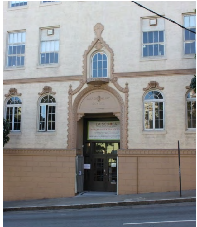
FIGURE 44. SCHOOL: MAIN ENTRANCE, 2015.
