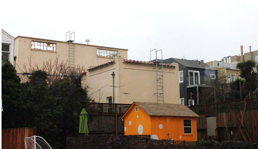
FIGURE 51. CONVENT: REAR (NORTH) ELEVATIONS OF CHAPEL ELL AND MAIN BLOCK, 2016.
