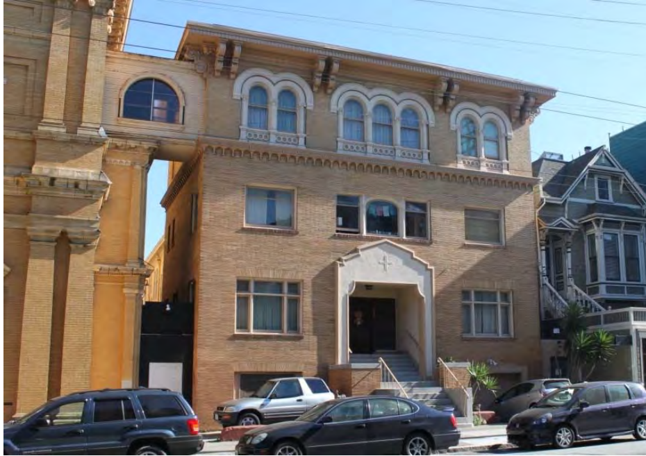
FIGURE 38. RECTORY: MAIN (WEST) ELEVATION FROM FILLMORE STREET, 2015.
