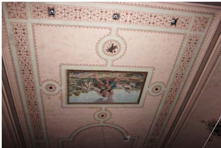
FIGURE 29. CHURCH: NAVE, WEST PORTION OF PAINTED CEILING, 2016.
