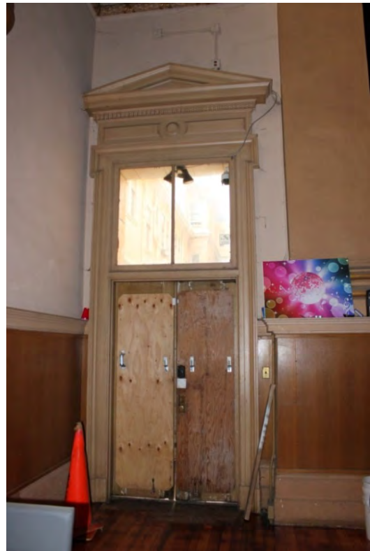
FIGURE 31: CHURCH: NAIVE, SOUTH TRANSEPT ENTRY TO ALLEY, 2016.
