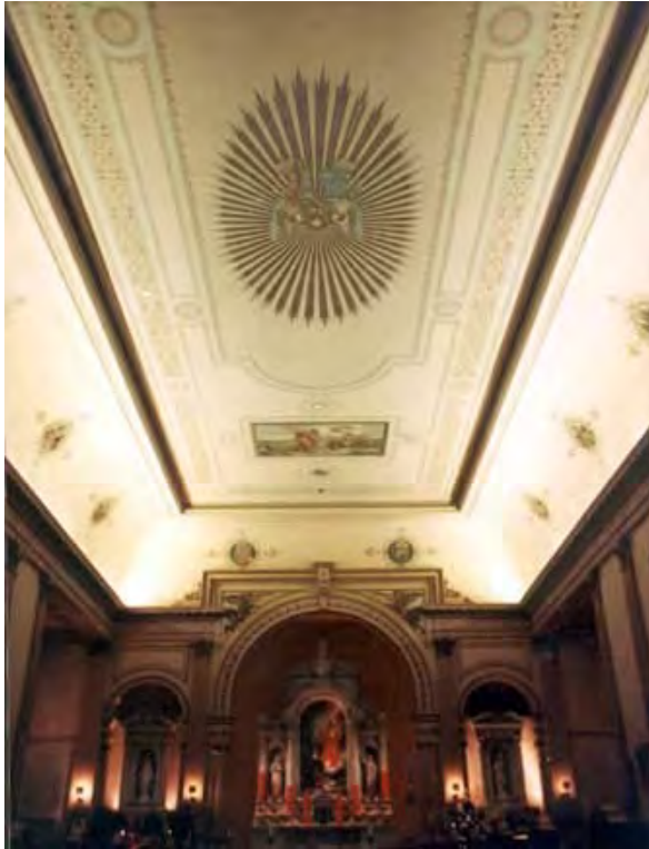
FIGURE 27. NAVE CEILING BEFORE HANGING OF SAFETY NETTING IN 1989 (PHOTO 2005, COURTESY KATHERINE PETRIN).
