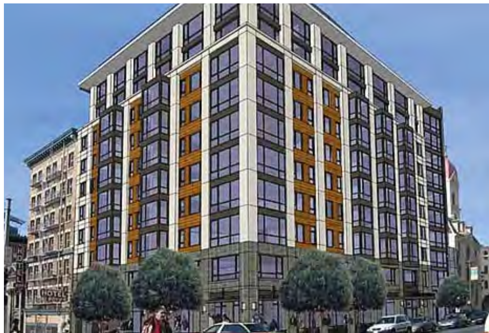
4. ST. ANTHONY'S BUILDING CURRENTLY UNDER CONSTRUCTION
