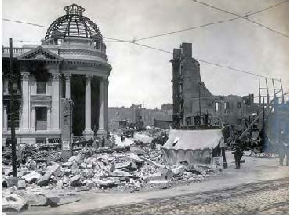
Source: HANCOCK LAMBERT, U.C. DUMAS 1. VIEW FROM MARKET STREET, AFTER FIRE / CIRCA 1906
