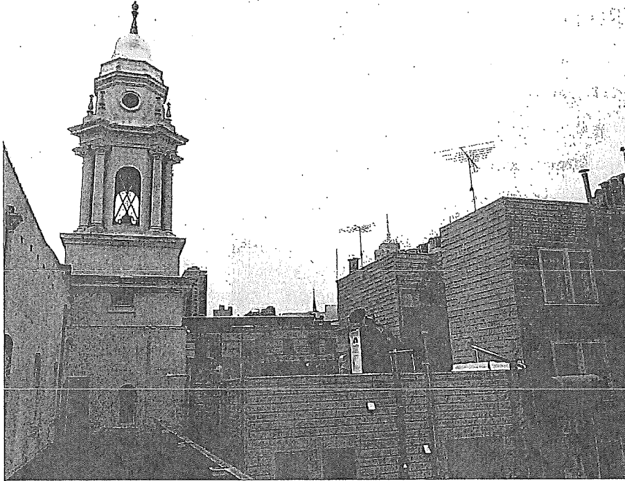
Twin tower on western portion of building exterior, view south.
