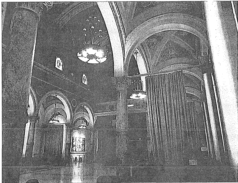
Interior view of sanctuary, view southeast.
