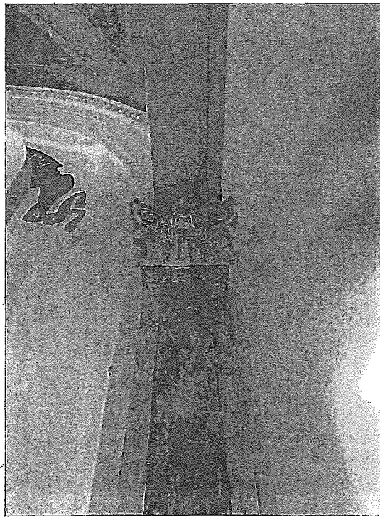
Detail of Corinthian pilaster.
