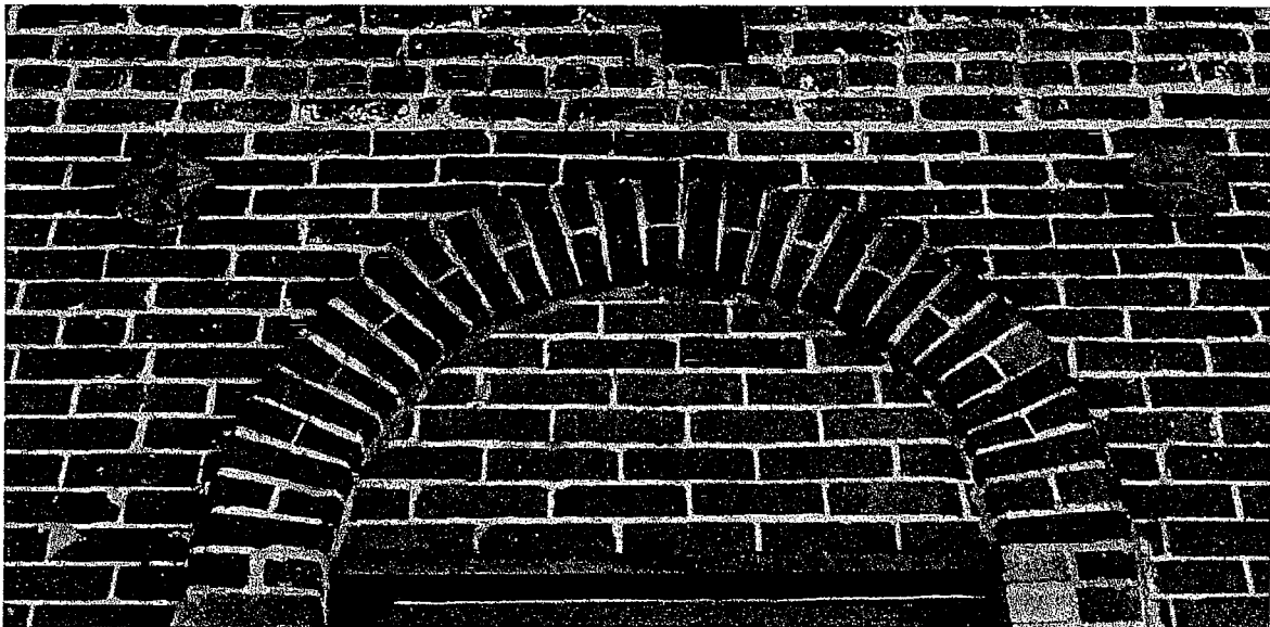
Figure 102 Detail view of pin holes left in brick tympanum over westernmost door along Vallejo Street (photograph taken on 03/30/2017).
