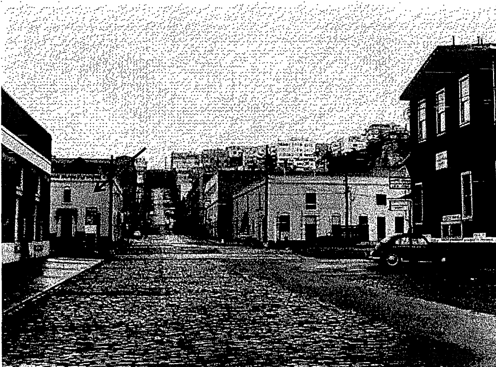
Figure 2: Vallejo Street, looking west from Davis Street (1962). Arrow pointing to 101 Vallejo: the Trinidad Bean and Elevator Co. Source: San Francisco Public Library, Image #AAB-5646. Edited by Page & Turnbull.
