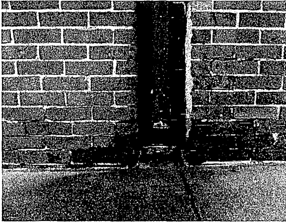
Figure 34 Non-functioning downspout along Vallejo Street. The inability to direct water away from the facade and foundation have resulted in heavy areas of bio-colonization. This will, in turn, accelerate the deterioration of the brick and mortar (photography taken on 03/31/2017).
