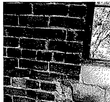
Figure 86 Detail of typical brick condition for deteriorated bricks around window openings (photography taken on 04/04/2017).
