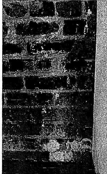
Figure 63 Detail of Portland cement patch and subsequent crack as a result (photography taken on 04/10/2017).
