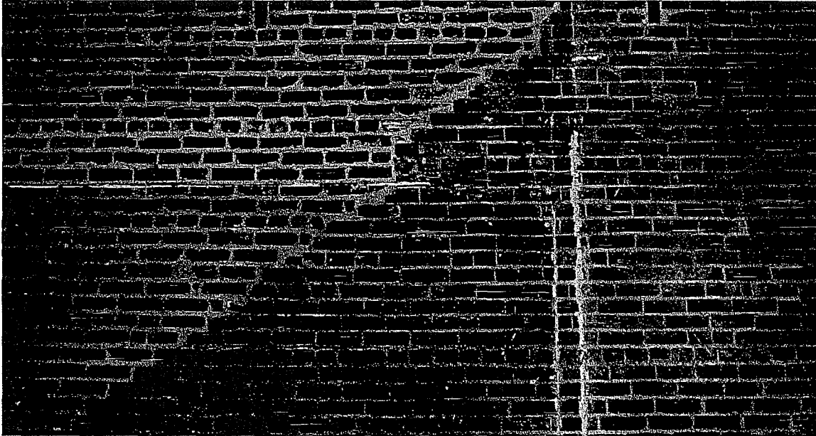
Figure 67 Photograph of south wall at the ground level. Note distinctively different eras of brick and mortar (photography taken on 04/04/2017).
