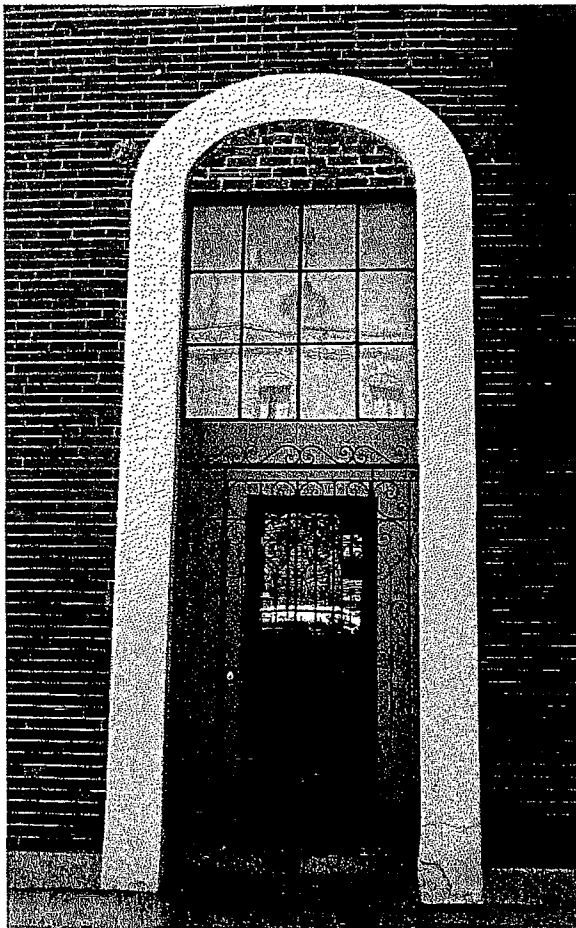
Figure 19 Photograph of easternmost entrance on Vallejo Street (photography taken on 03/30/2017).
