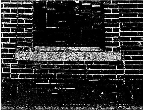
Figure 32 Detail of biological colonization plaguing mortar joints at the bottom courses along Vallejo Street (photography taken on 03/31/2017).
