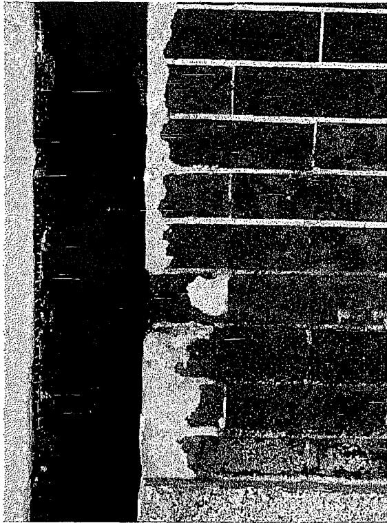
Figure 91 Detail view of incompatible repair along Front Street. Note dissimilarities between brick and repair, and note bio-colonization plaguing the joints (photograph taken on 03/31/2017).
