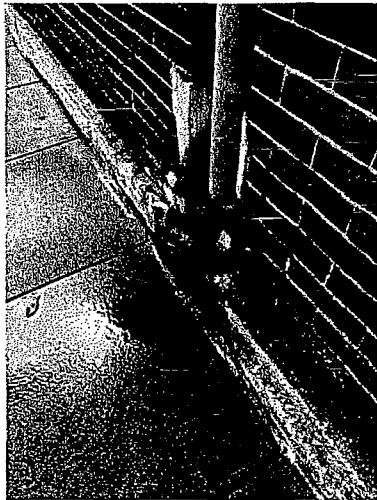
Photo 23: Outlet of downspout at sidewalk.
