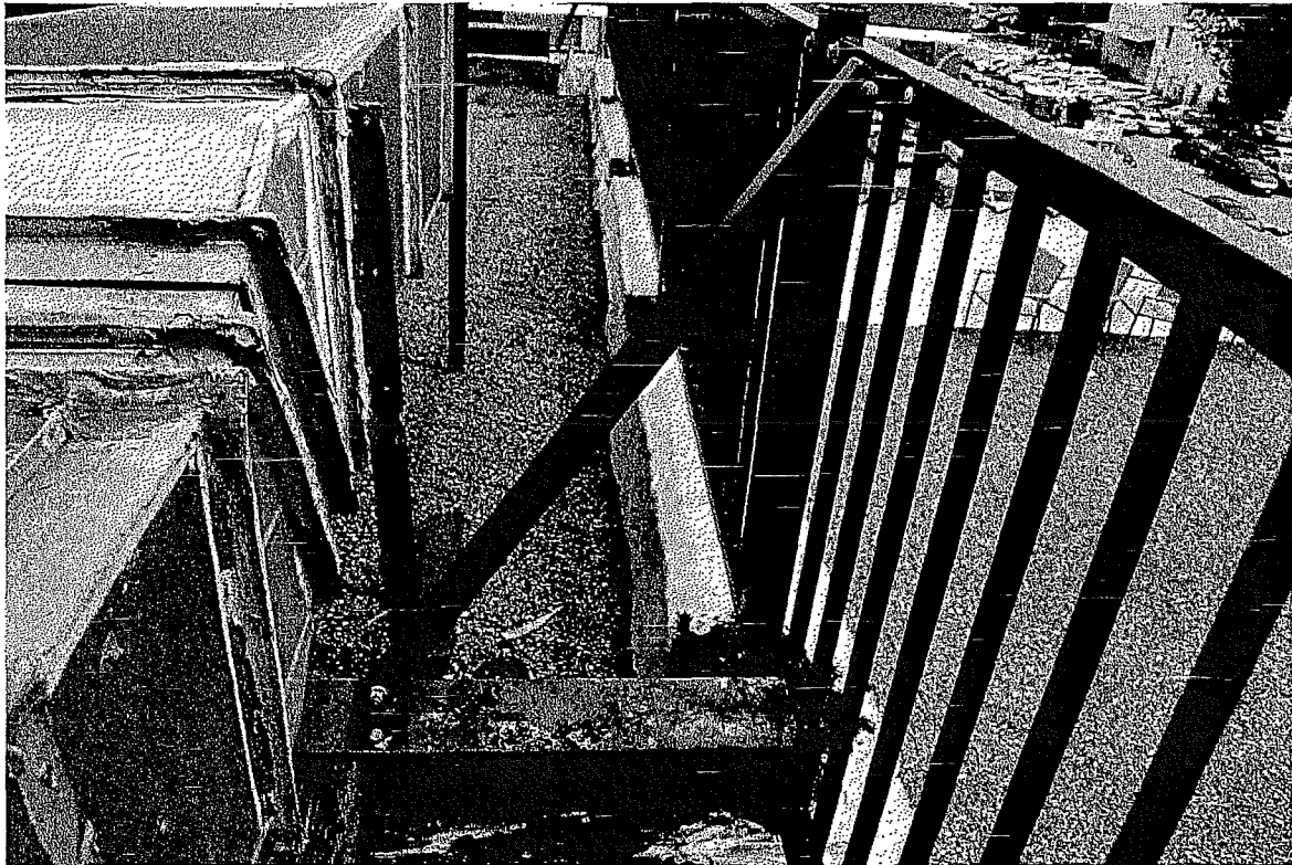
Figure 55 Photograph of non-historic railing and construction (photography taken on 04/04/2017).
