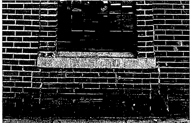
Figure 29 Detail of biological colonization at the bottom courses along Vallejo Street (photography taken on 03/31/2017).
