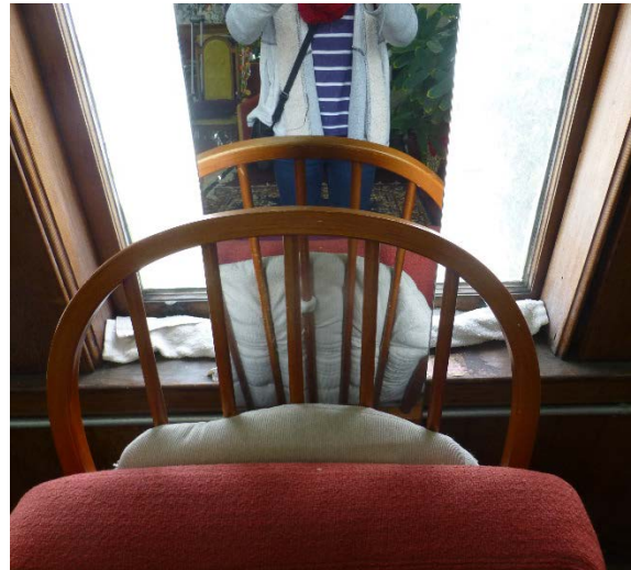
Figure 30: Window covered by long mirror and inadequately weatherstripped with a towel.
