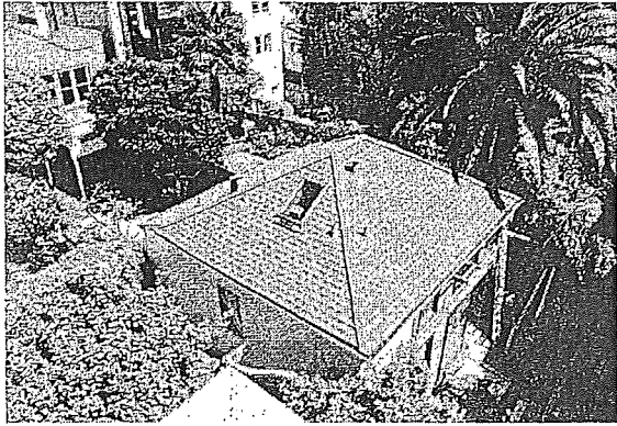
Figure 14. Cottage at rear of 20 Beaver Street.
