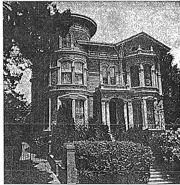
Figure 55. Coleman-Wormser House, 1834 California Street, 2017. Source: Google Maps
