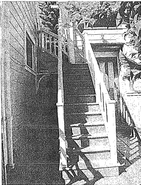
Figure 23. Patio and stair; view toward west.
