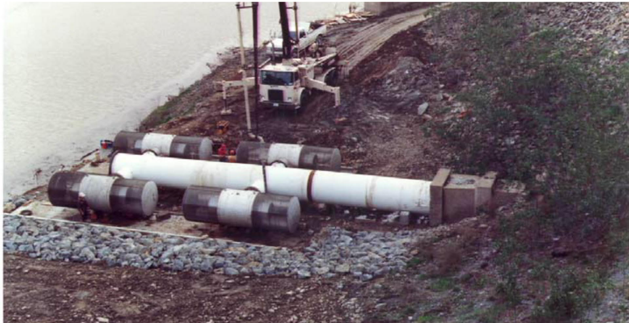
Figure 7-2: Completed Intake Screens on Open-Water Intake Tunnel
