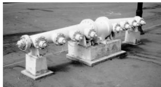
Figure 2-5: Typical Fireboat Manifold Inlet
