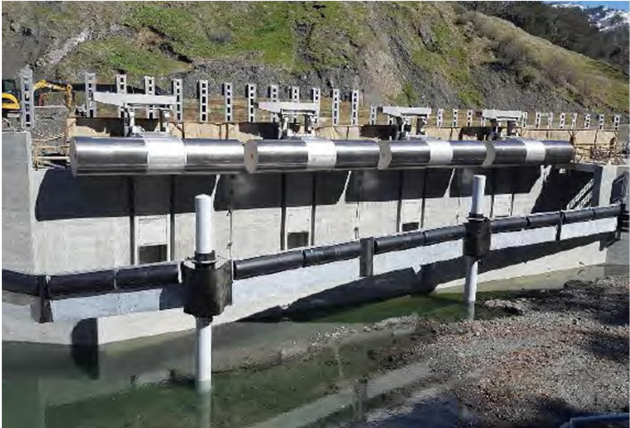
Figure 7-3: Intake Screens at Alameda Creek Diversion Dam
