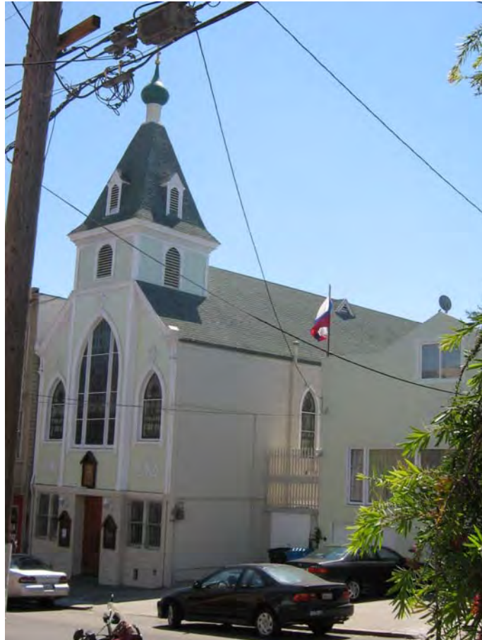
View from the northwest
