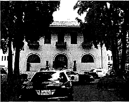
SFPD Park Station
