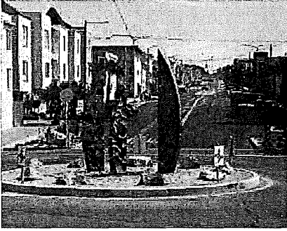
Recently Completed Taraval Streetscape Project
