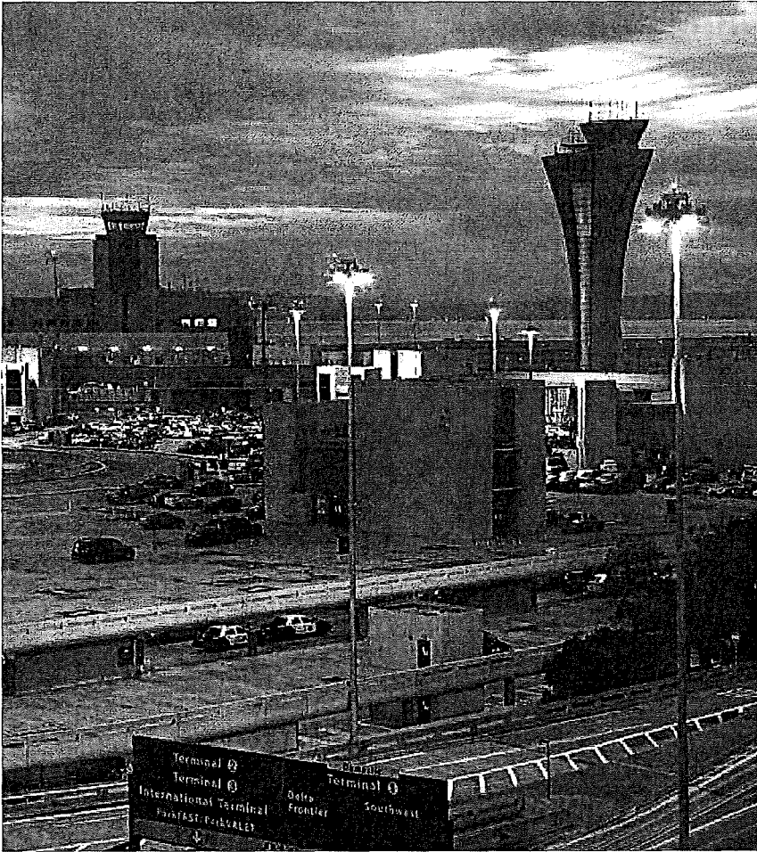
New Control Tower at SFO
