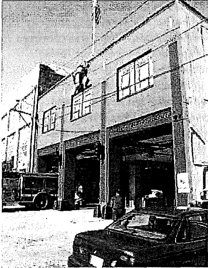
SFFD Fire Station
