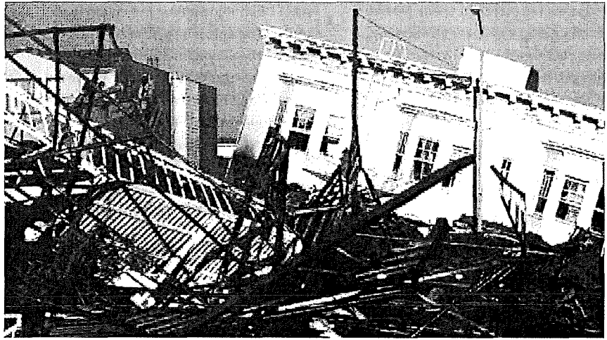
1989 Loma Prieta Earthquake
