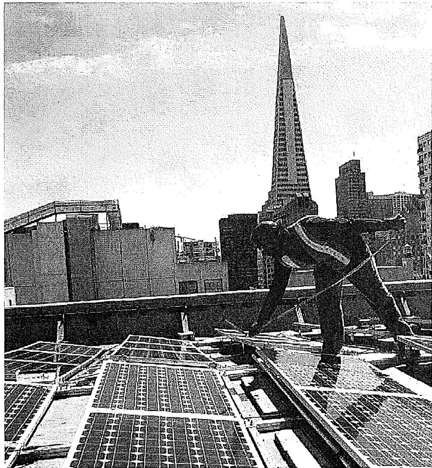
Solar Panel Installation at City Facilities
