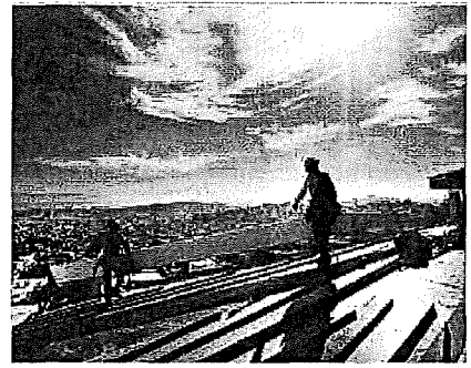
New Roof at the Ashbury Tank
