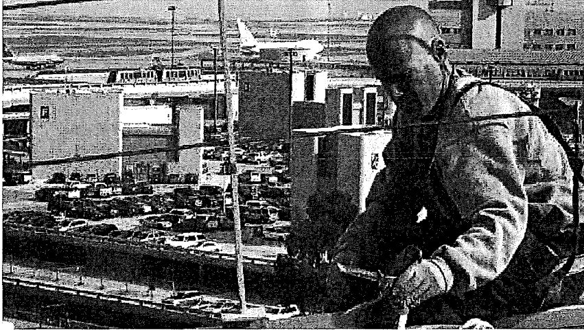
Roof Repair at SFO
