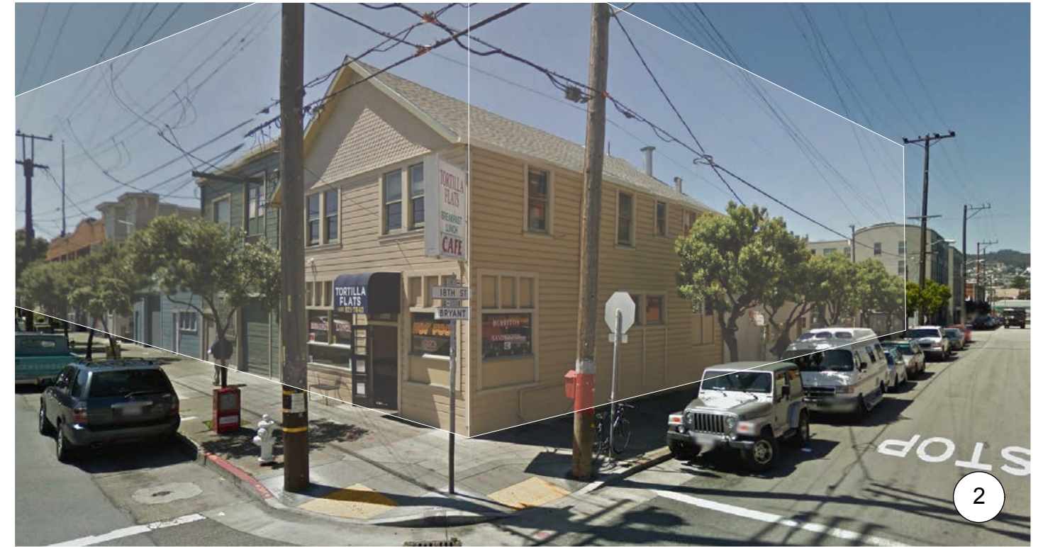
18TH STREET: VIEW WEST DOWN 18TH
