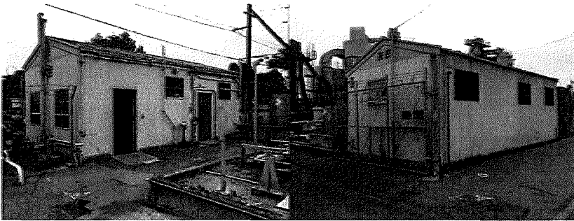
Women's Restroom/Locker Room. Southwest facing elevations (left), and northeast facing elevations (right)
