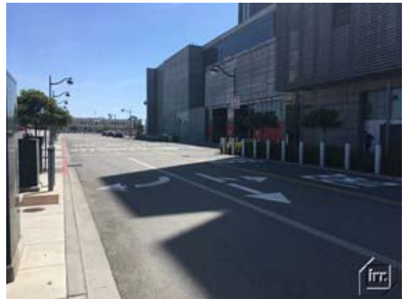
Mission Rock Blvd – Facing East
