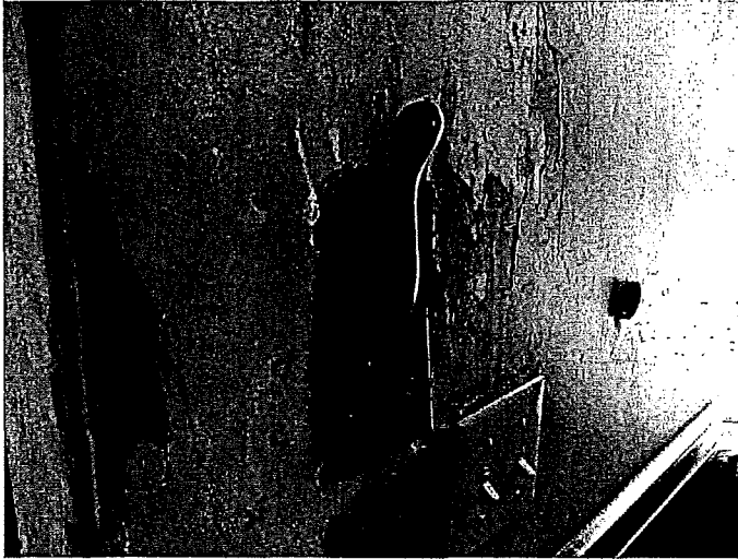
Figure 29 The bronze handle and speaking-horn at the top of the stairwell at 194 Gough Street is unlike Rube Goldberg's elaborate machinations that accomplished a mundane task with great effort. These devises allowed him to communicate with the person at the front door downstairs and to pull the lever to open the door if they are welcomed guests without having to descend the steps himself.
