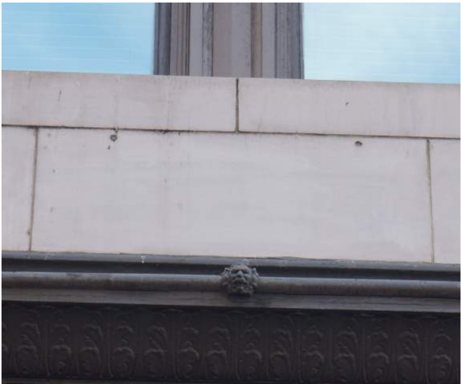
Hearst Building – Minor previously patched holes mismatched with surrounding terra cotta glaze
