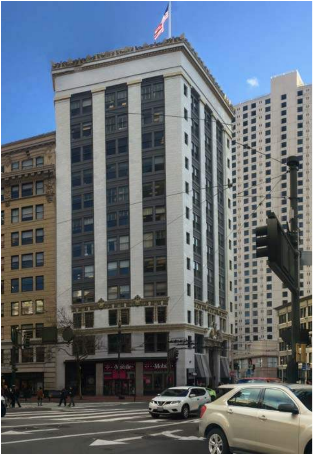
EXISTING view looking southeast from Market Street
