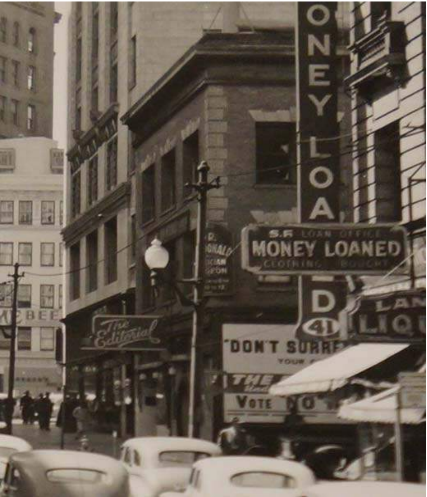
Storefronts at Third Street, October 1946
