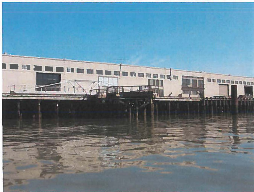
Photo 2. Exterior view from the South
