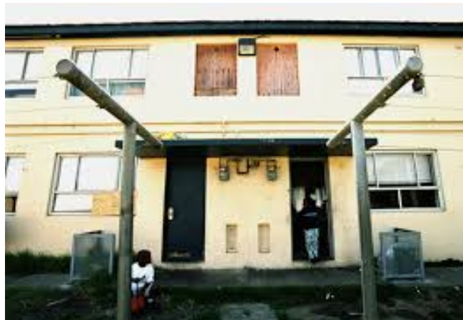
Hunters View public housing before HOPE SF transformation
