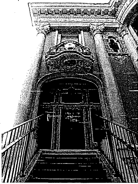
Figure 14: Molded balcony with flanking engaged columns.
