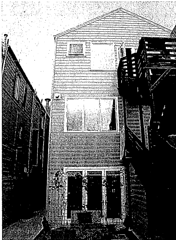
Figure 29: South side fenestration.
