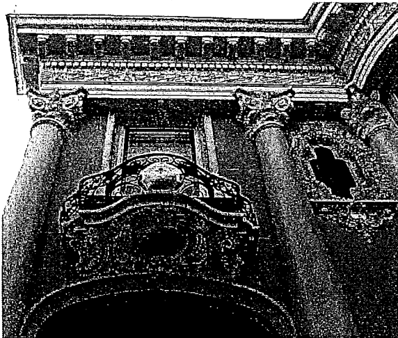
Figure 16: North side of primary façade.
