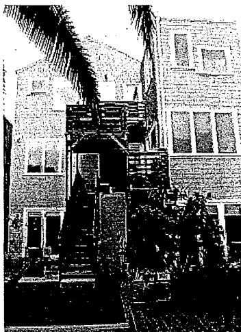
Figure 25: Rear (east) façade with south (left) and north (right) sides.
