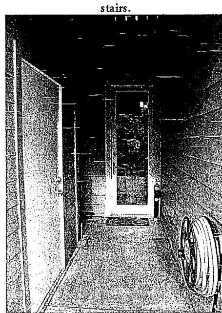
Figure 28: Storage door and south façade access door.
