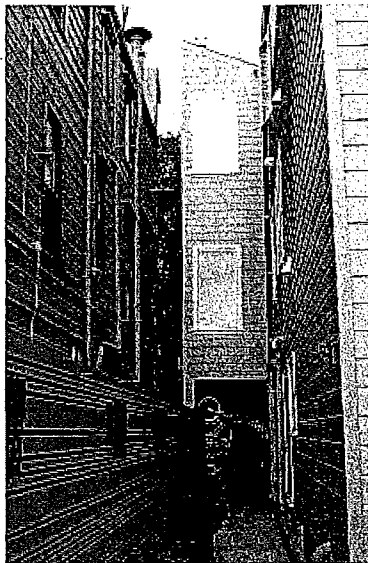
Figure 22: South façade with projection and passageway, view facing west.
