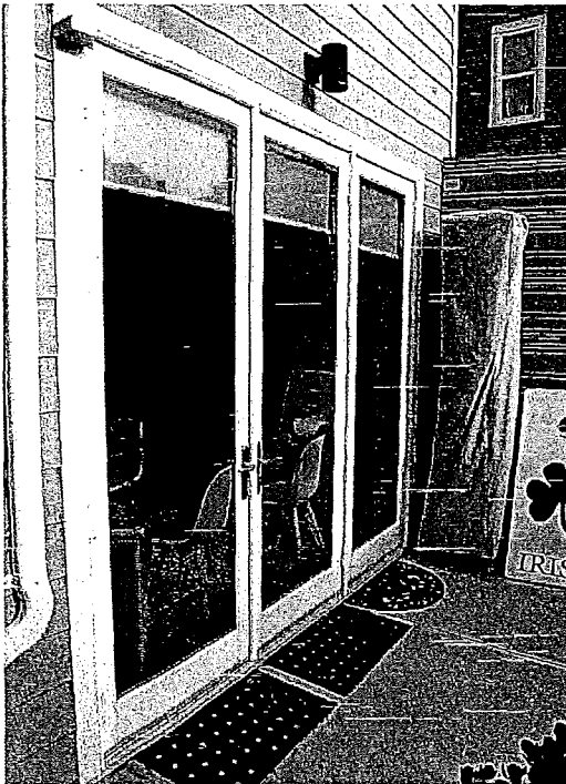
Figure 31: North side ground level.
