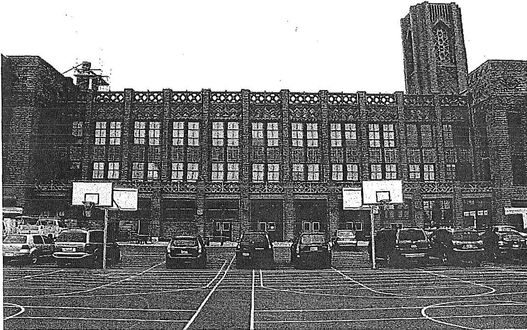
Figure 29. Central section of east façade of Theodore Roosevelt Middle School; view toward west.
