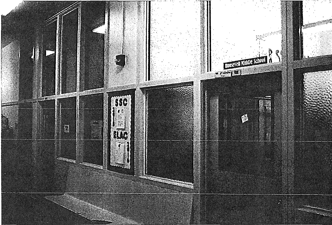
Figure 47. Windows and bench in administration office suite.
