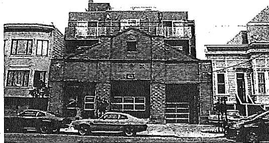
Figure 5. 421 Arguello Boulevard, built 1912 and 2012; view toward west.
