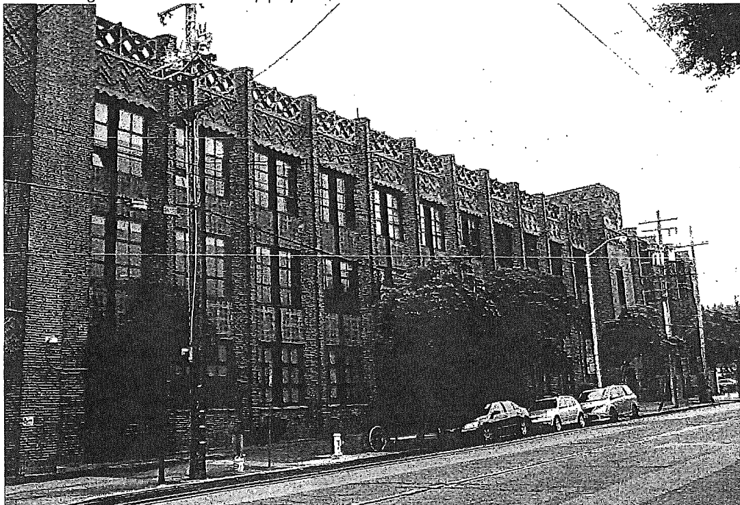
Figure 23. Academic building; view toward southeast.
