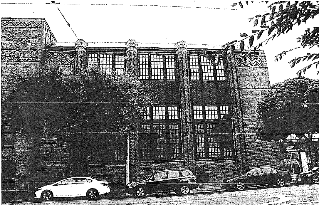
Figure 26. West façade of gymnasium wing.
