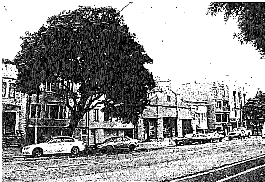
Figure 4. West side of the 400 block of Arguello Boulevard; view toward northwest.
