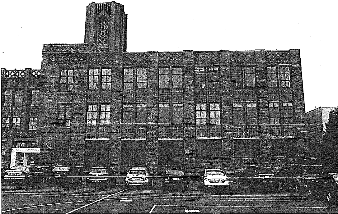
Figure 30. North section of east façade of Theodore Roosevelt Middle School; view toward west.
