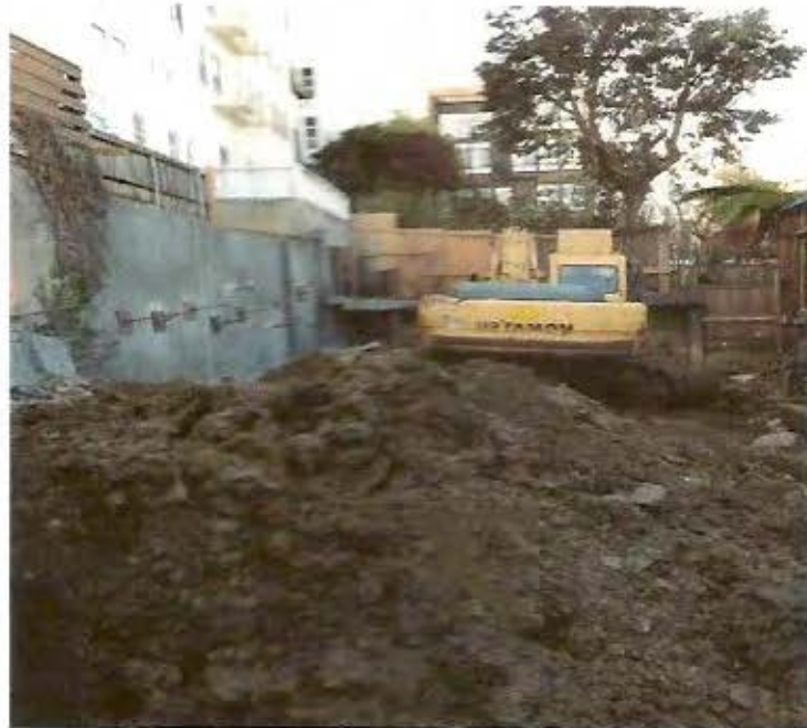
Ties Backs in Consolidated Larkin Retaining Walls
