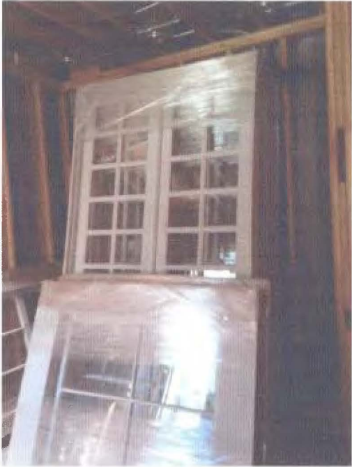
Main doors of the Studio ready for installation, April 2014
