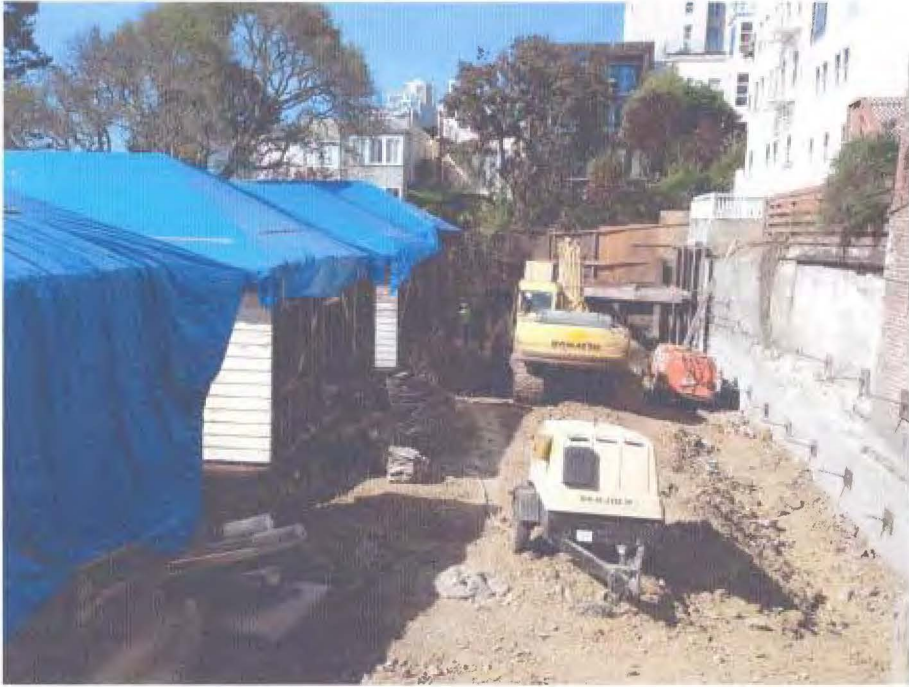
Cottages shored and cribbed during Rehabilitation
