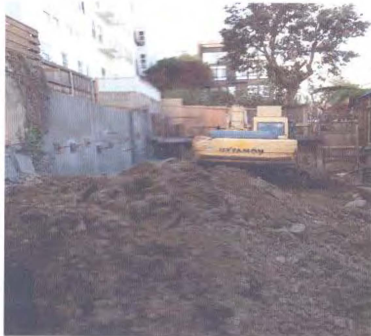
Ties Backs in Consolidated Larkin Retaining Walls
