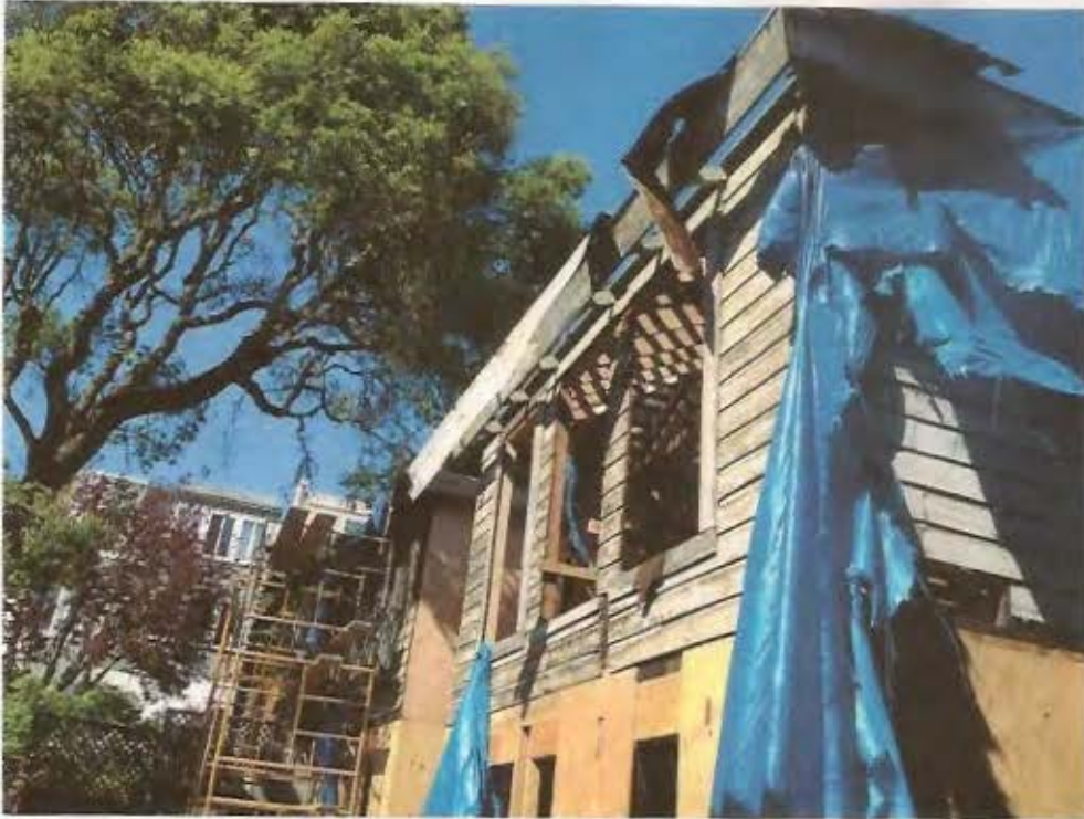
Shoring during Rehabilitation
