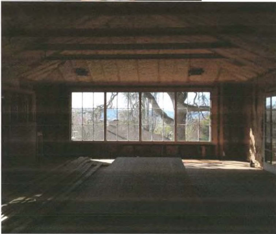
Restored entry door and window in unit D, April 2016
