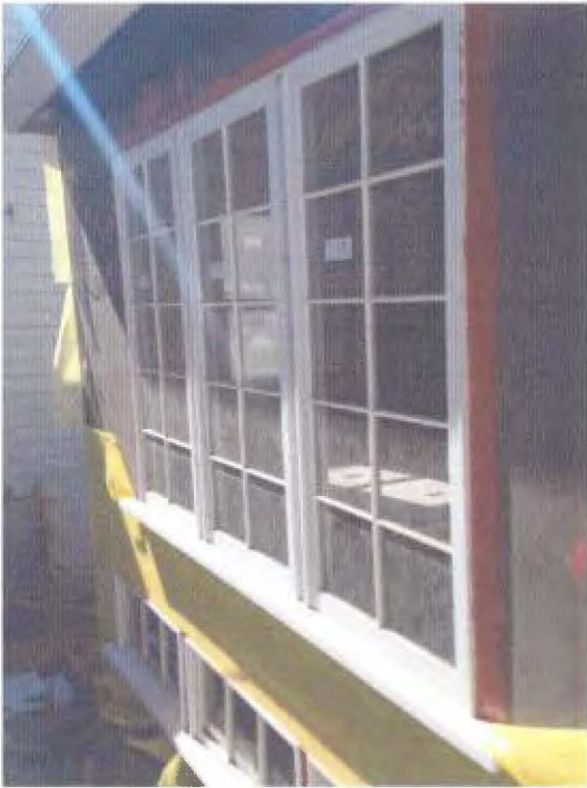
South Façade of Cottage A waiting for siding, April 2016
