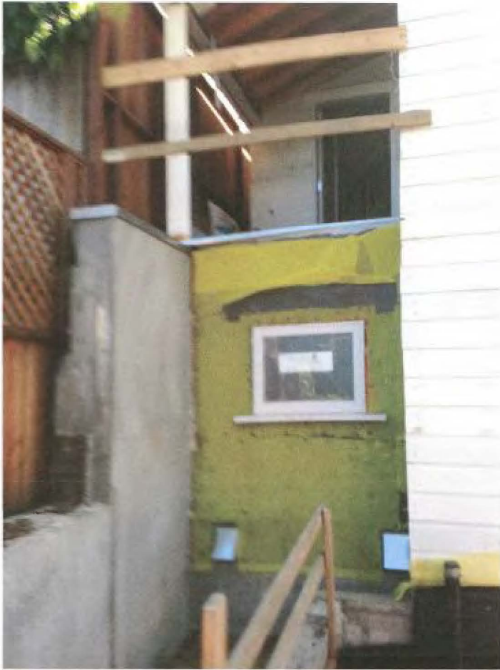
Cottage D, exterior before stairs, April 2016
