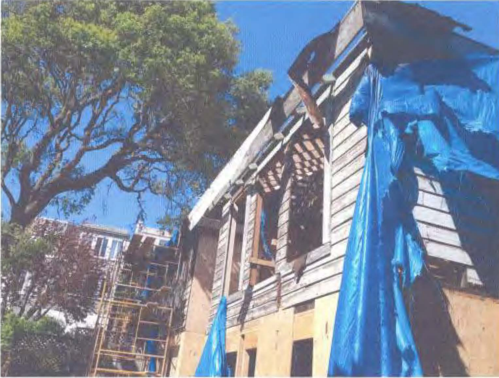
Shoring during Rehabilitation
