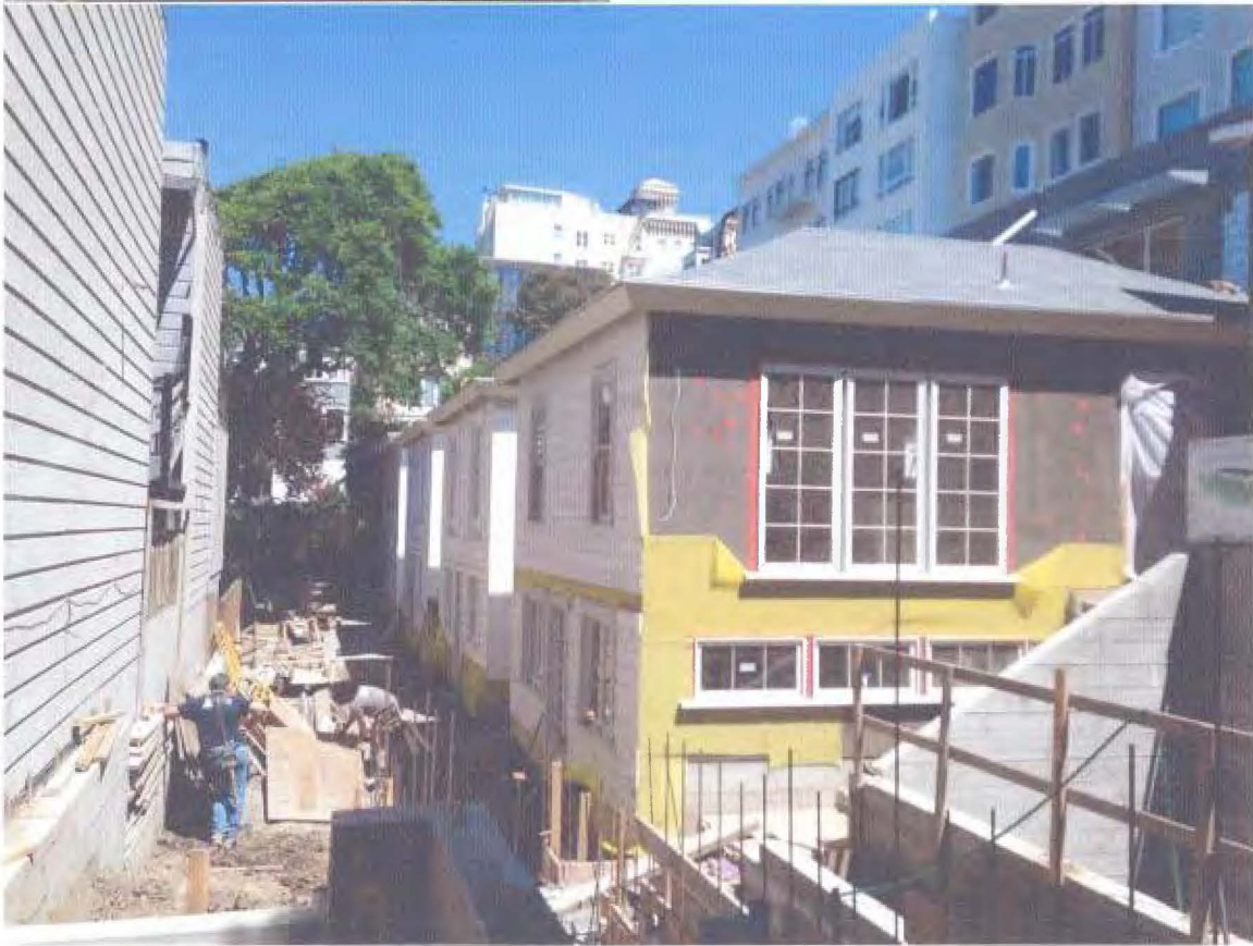
View from the street Cottages A through D, April 2016
