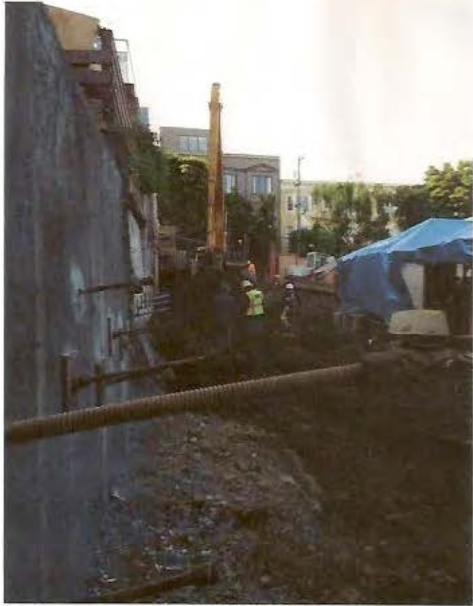
Ties Backs in Consolidated Larkin Retaining Walls
