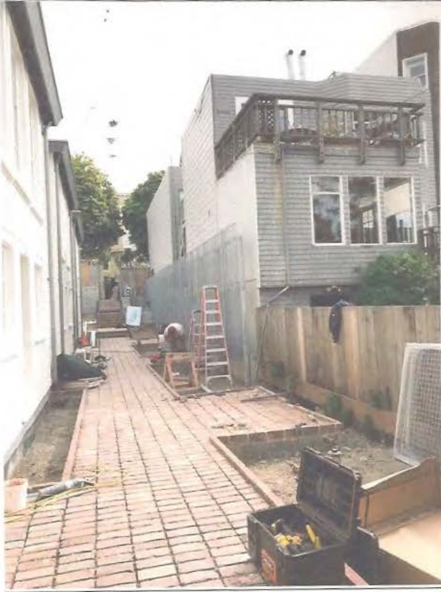
Pictures of 1338 Filbert Street in 2017, showing final restoration of the roofs, brick pathways, the siding and painted cottages, the grape stake fence and the planting of the Garden:
