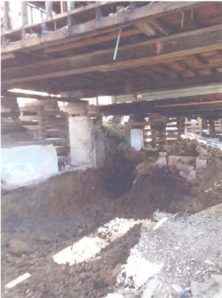
Cottages shored and cribbed during Rehabilitation
