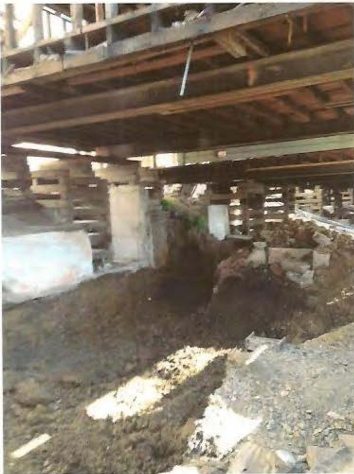
Cottages shored and cribbed during Rehabilitation
