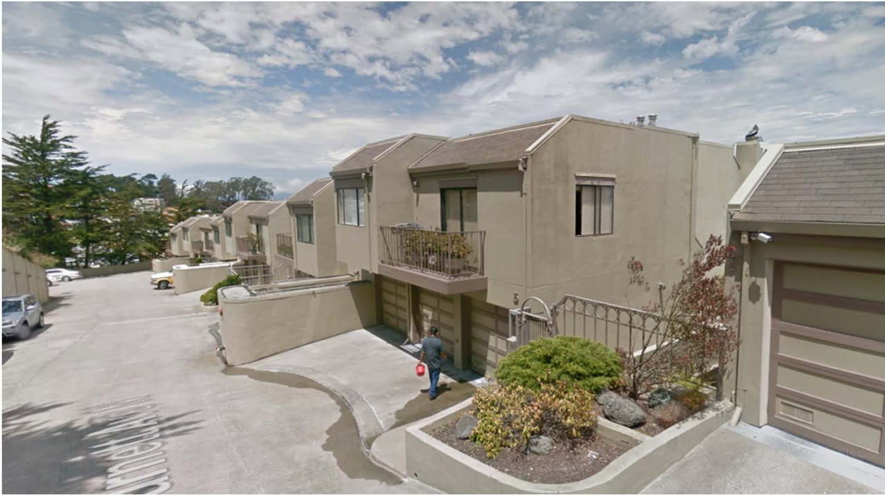
1 – 20 Burnett Avenue North is a condominium complex with one story over a garage at the street and contains four floors to the rear.
