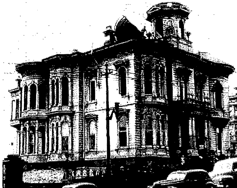
Above: Workers remove the turret on the observatory in the cupola of the former mansion of Captain Charles Goodall at Pierce and McAllister Streets, which was demolished and replaced with Third Baptist Church in 1952 (Courtesy San Francisco Public Library Photo Collection)
