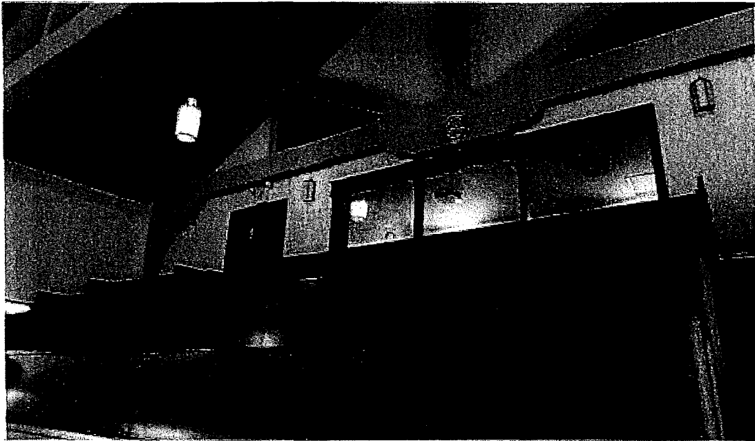
Mezzanine. View northwest.
