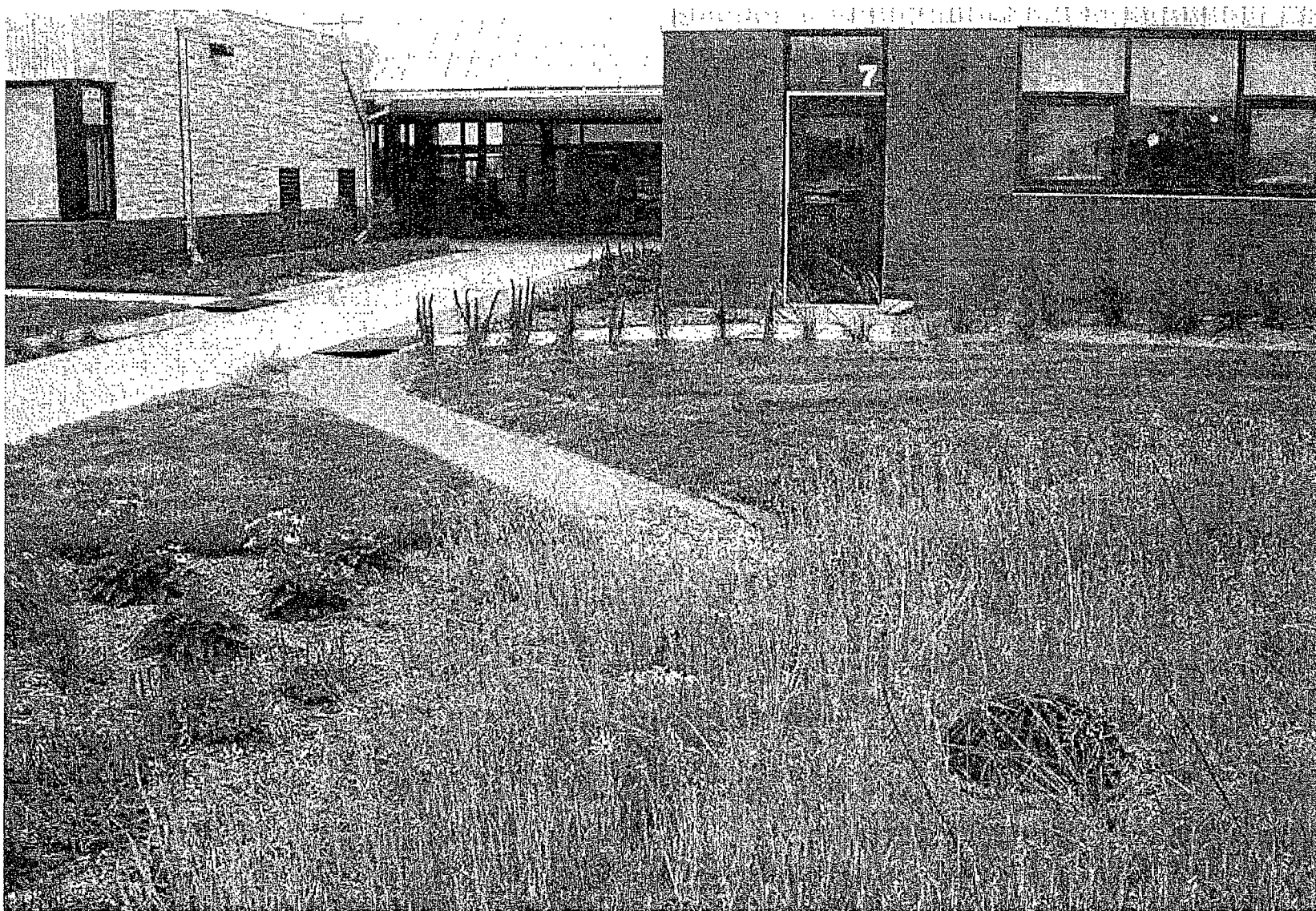
An impervious gutter directs roof runoff to a rain garden. Photo: Ken Kortkamp
