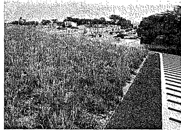
The vegetated roof at the Ortega Branch Library in San Francisco includes an Ortega Living Roof Cam that streams on their website. Photo: Robin Scheswhol
