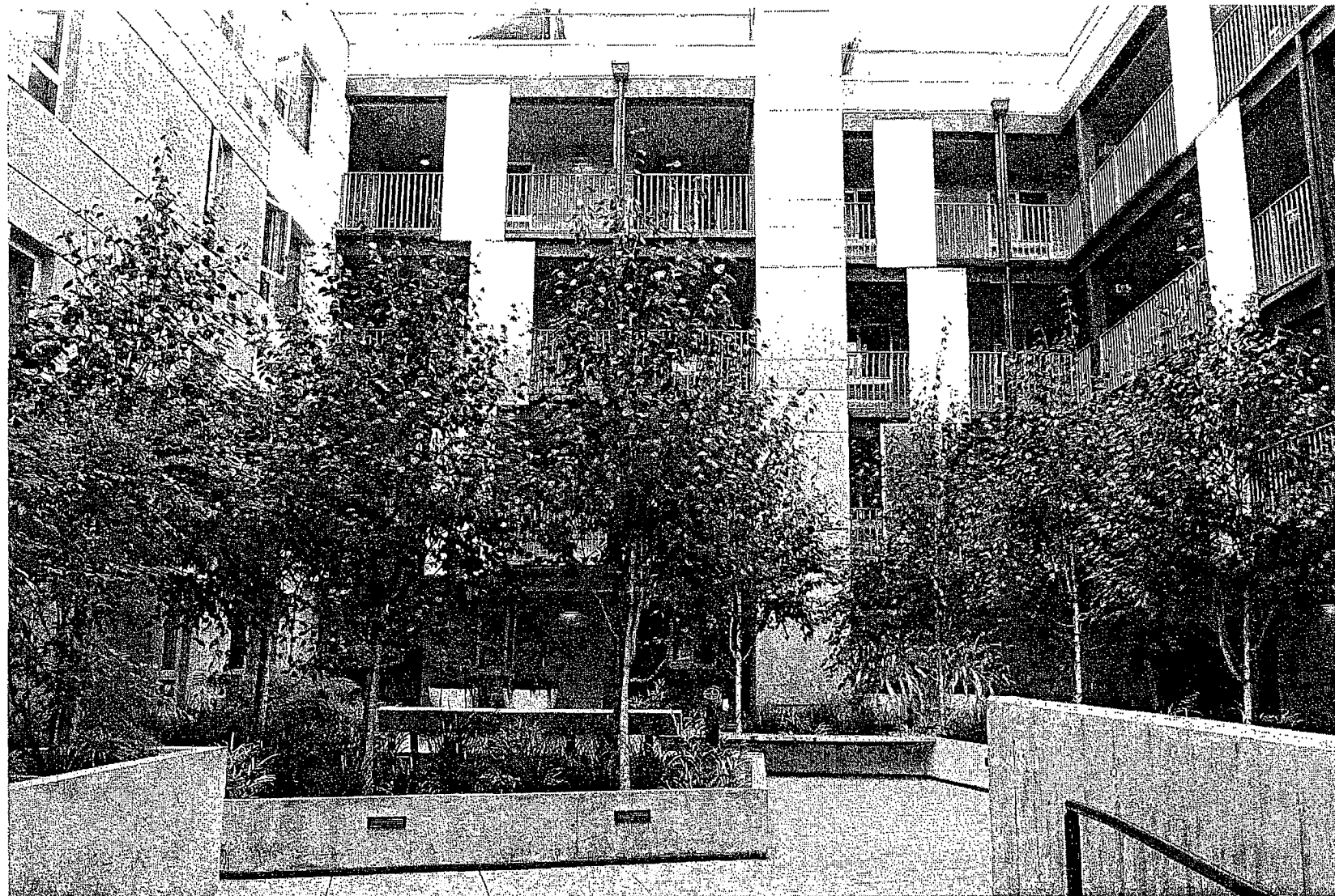
Bioretention planters are a central fixture in a courtyard area. Photo: Krystal Zamora
