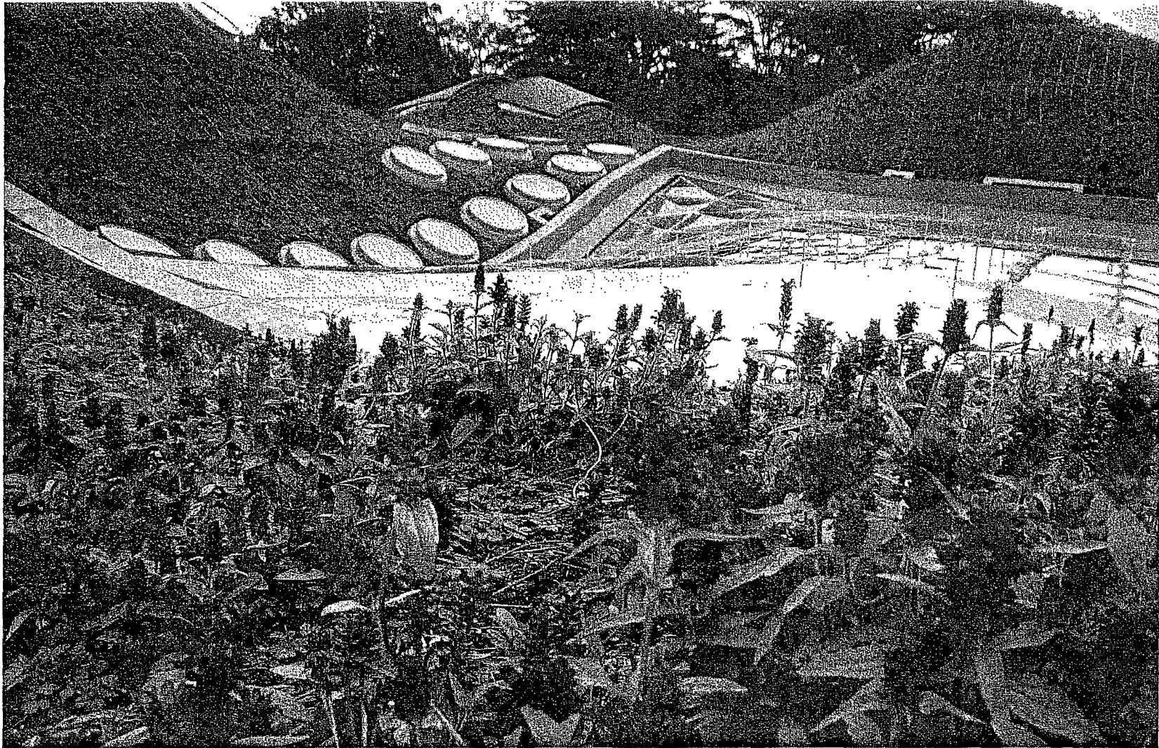
The Academy of Sciences in Golden Gate Park is a LEED Platinum building and includes a 2.5-acre vegetated roof. Photo: Rana Creek — Living Architecture
