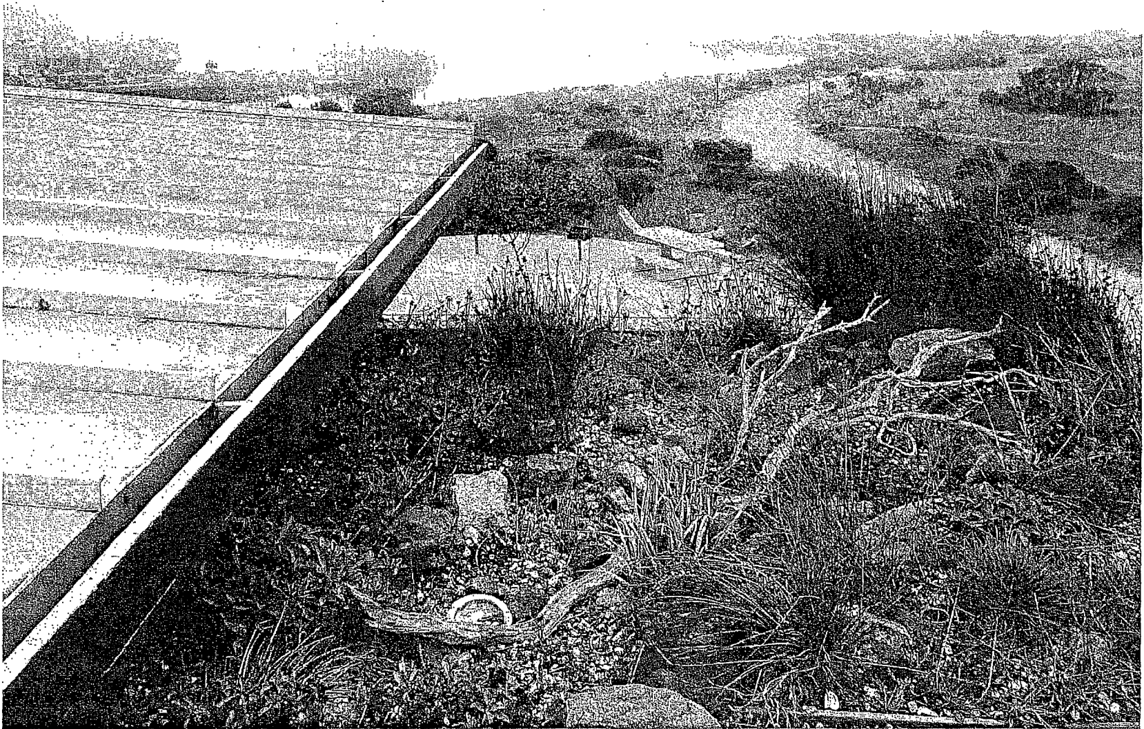
A vegetated roof and other LID features at the Eco-Center at Heron's Head Park help illustrate sustainable design practices to students in San Francisco's Bayview-Hunters Point neighborhood. Photo: Rosey Jencks
