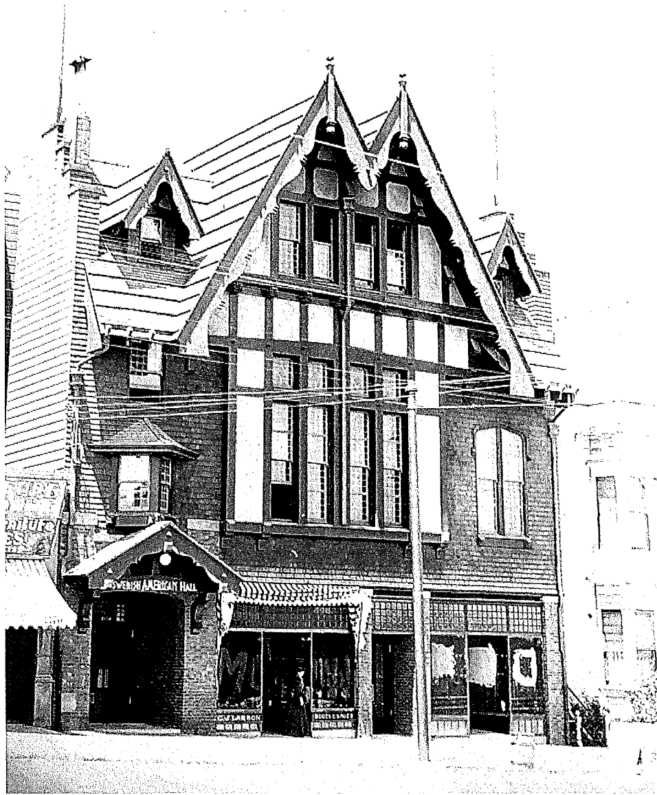
The Swedish American Hall, ca. early 1908. Note that the storefront at 2168 Market Street is still under construction. (Ted Olsson Collection)
