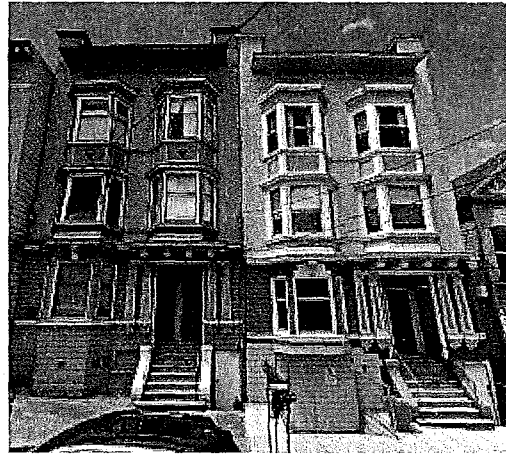
Flats at 847-851 and 853-857 Cole Street designed by August Nordin and completed ca. 1904. 23 (Google Maps)
