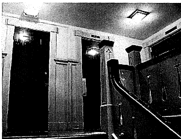
Second floor landing. From left to right a closet, men's room and double doors leading to the Freja Hall ante room. Both the closet and men's room were removed in 2014 to install an ADA compliant elevator.
