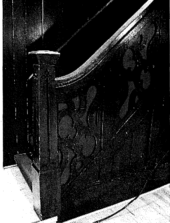
Detail of stair newel post and fretwork
