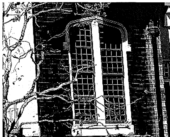
Detail of arched window
