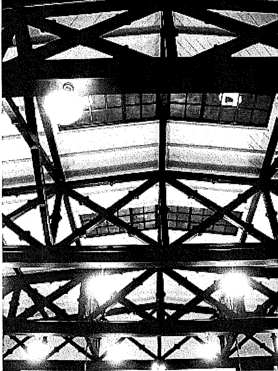
Detail of skylights
