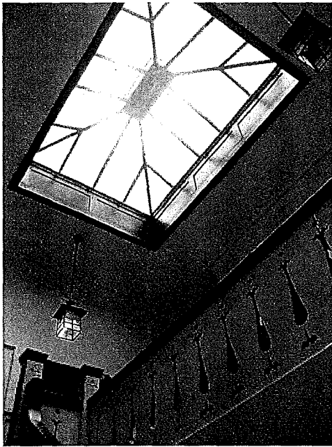
Detail of skylight above the third floor landing.
