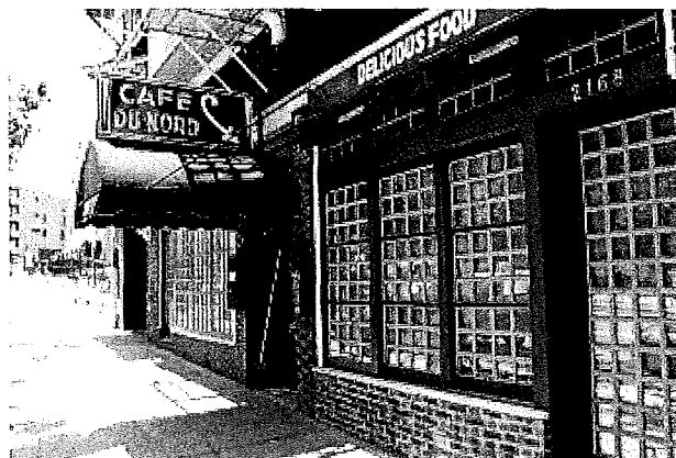
View of the storefronts. Note the non-historic brick cladding beneath the storefront window at right
