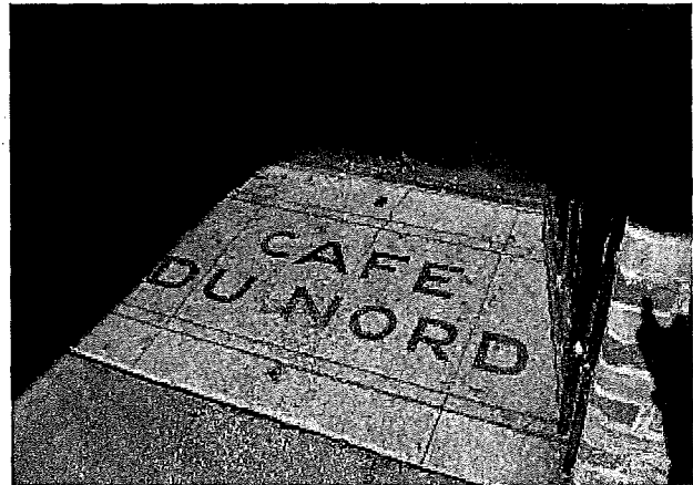
Detail of terrazzo threshold
