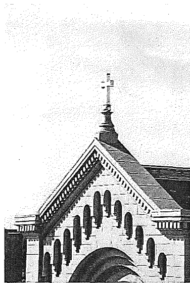
Figure 11. Detail of corbel table and cornice on the transept. Source: Rick Stapleton, September 2018.
