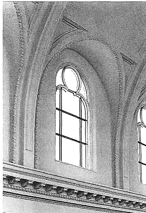
Figure 70. Typical clerestory window with protective glazing, interior view. (Rich Stapleton, 05/21/2018).
