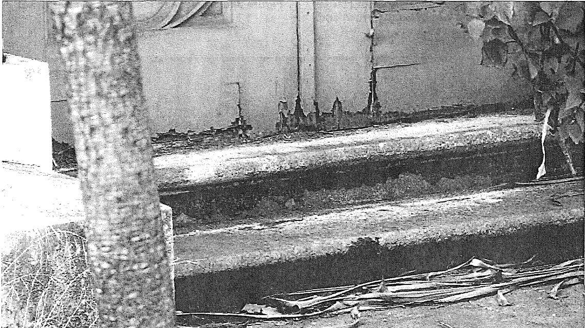
Figure 33c. East transept, north portal steps, showing decorative bull nose with biological growth and soiling.
