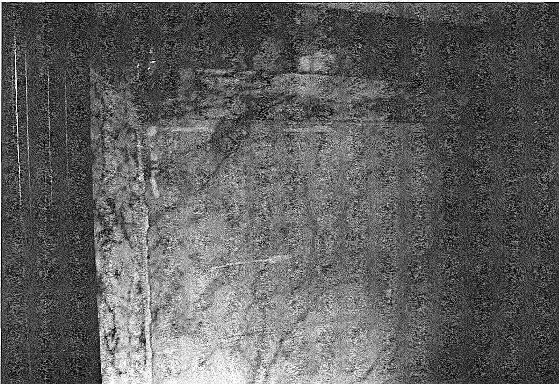
Figure 39b. Detail, showing tape and adhesive residue.
