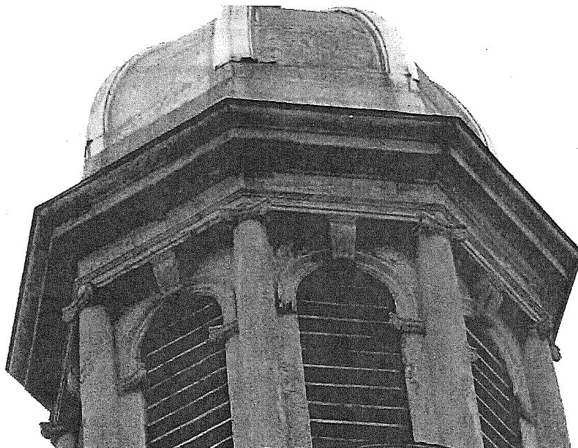
Figure 37c. East tower detail, constructed entirely of pressed sheet metal, showing missing architectural detail, loss of gilding and protective paint, and corrosion stains. Birds were nesting inside the towers.
