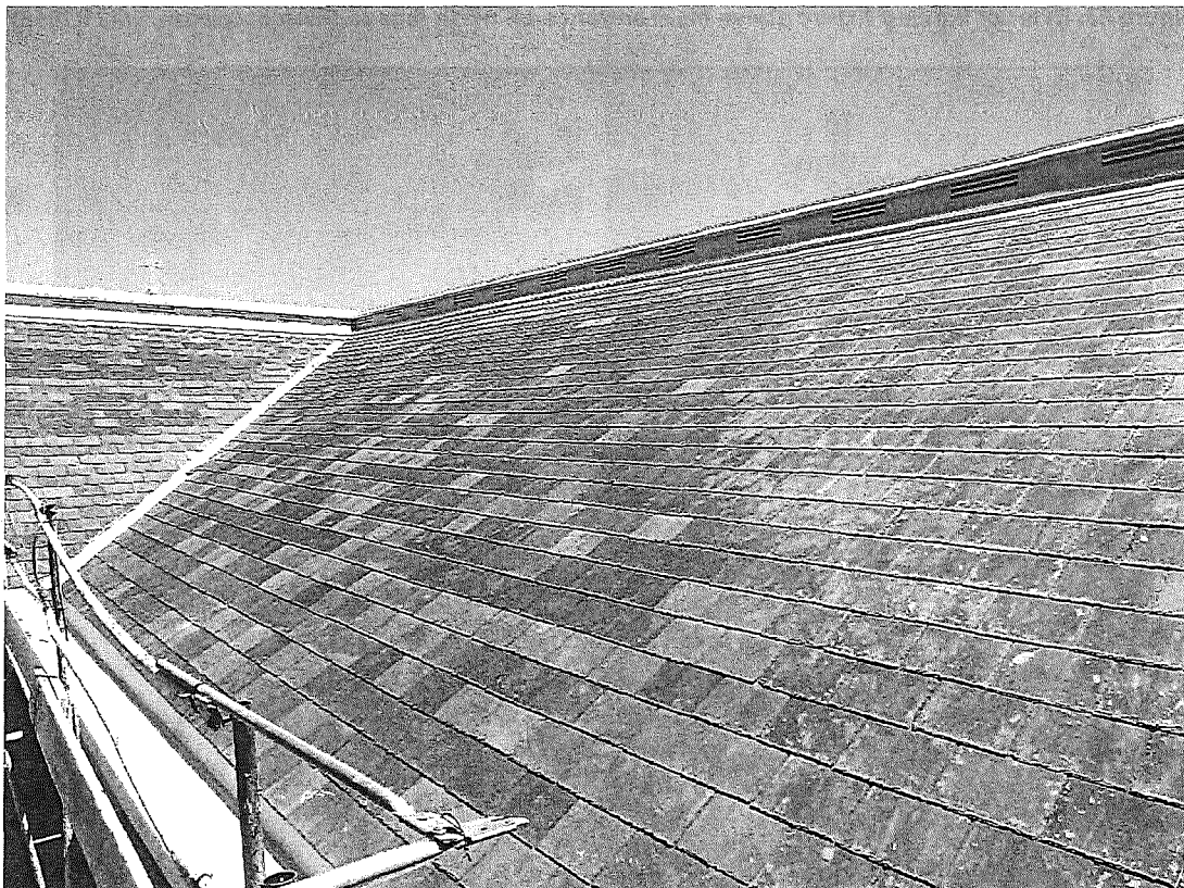
Figure 56. Main roof after restoration. (Palisade Builders, 05/20/2018)
