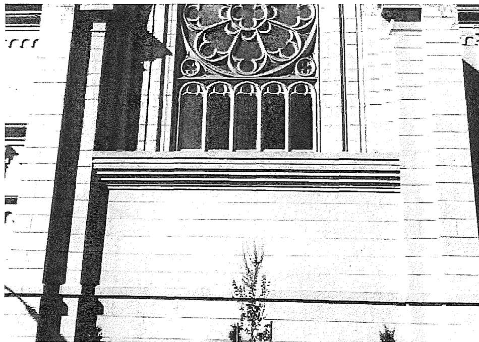
Figure 52. West façade, showing stucco condition after restoration (Page & Turnbull, 05/25/2018).
