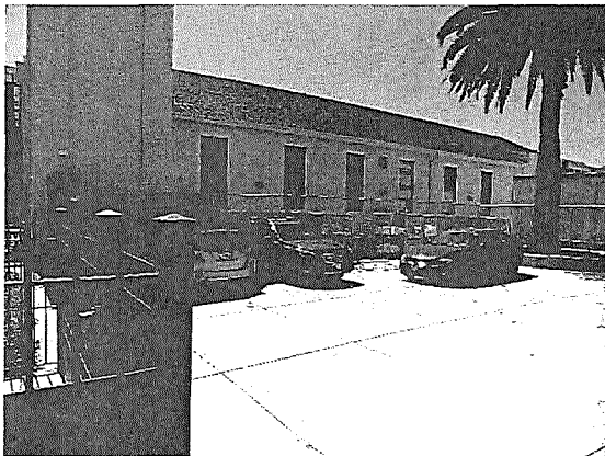
Figure 30. Concrete parking area southeast of St. Joseph's Church, at the former location of the garage, looking south.
