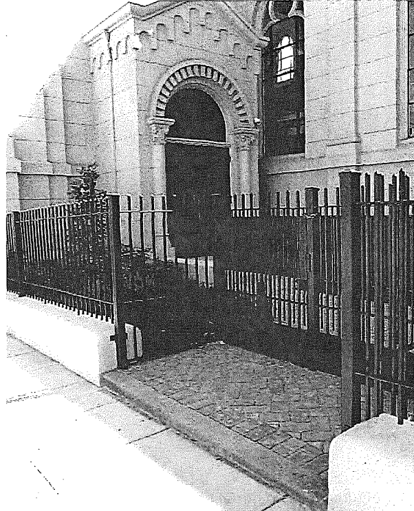
Figure 44. Perimeter fence and gate along 10th Street at the northeast corner of St. Joseph's Church. View southwest. (Page & Turnbull, 05/25/2018)
