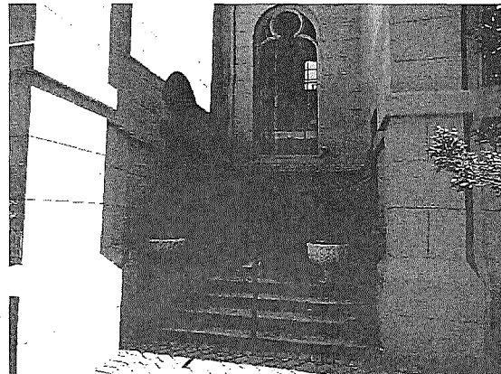
Figure 14. Recessed area between the west transept (left) and projecting bay (right).
