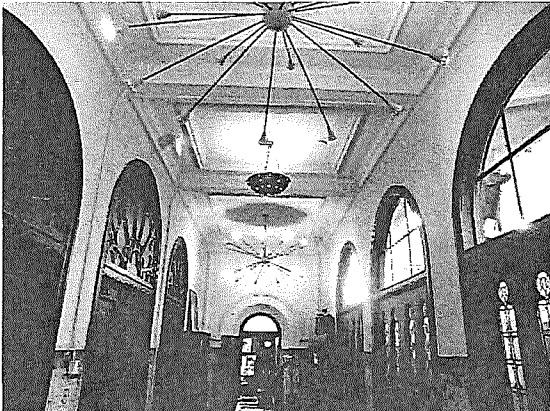
Figure 17. Narthex, looking east. Source: Page & Turnbull, April 2019.
