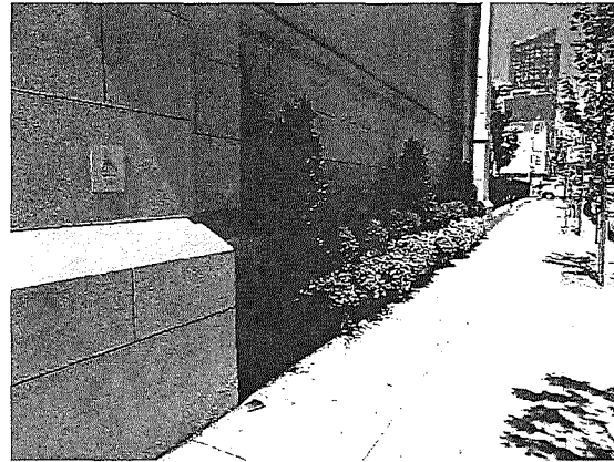
Figure 12. Contemporary steel planter at transept of east façade. Source: Page & Turnbull, April 2019.
