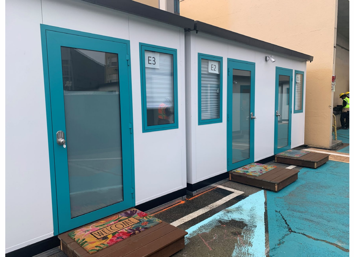
Non-congregate cabin at 33 Gough.
