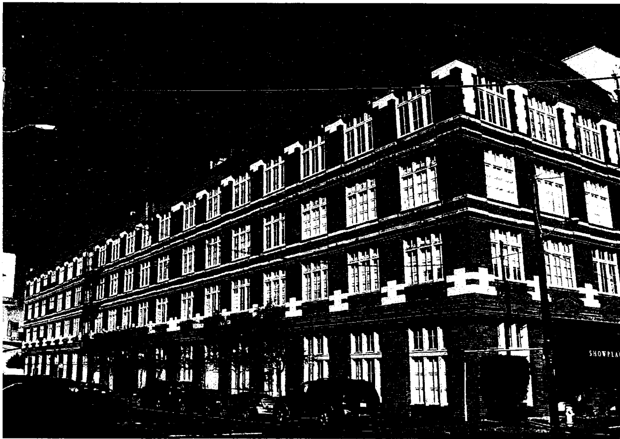
West facade (l), south facade (r)
