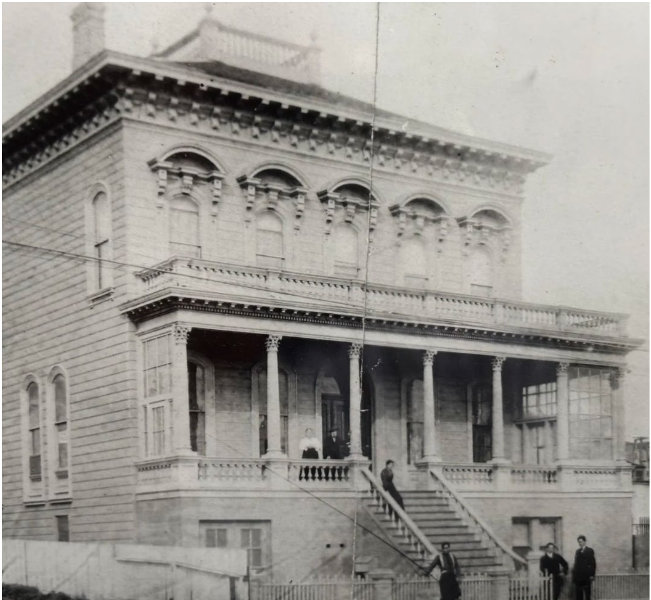
Blacketer-Sylvester House, 1556 Revere Avenue, front façade, view north, c. 1913. Source: The Sylvester House website
