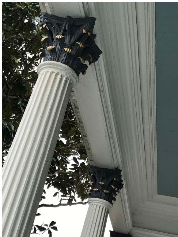
Blacketer-Sylvester House, 1556 Revere Avenue, fluted columns and cast-iron capitals, 2026. Source: SF Planning Department
