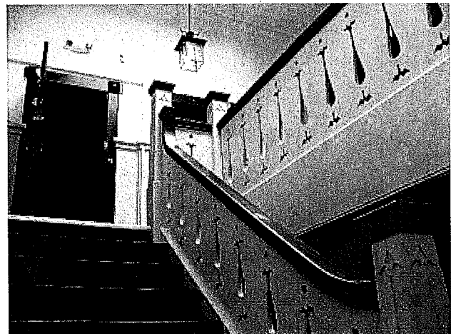
View from the stairs toward the third floor landing. The door accesses a closet since converted into an elevator shaft.
