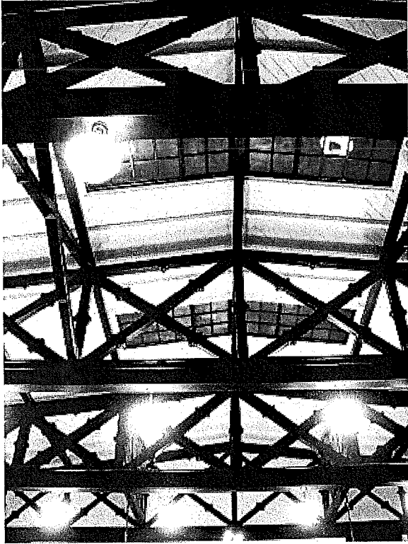
Detail of skylights
