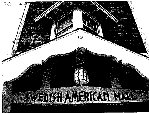
Gable hood above the main entrance to the hall
