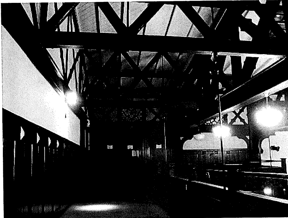
View west along the balcony. Note the metal bars which help suspend the balcony above the floor.
