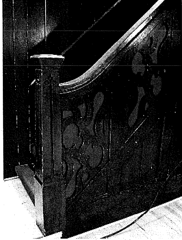
Detail of stair newel post and fretwork
