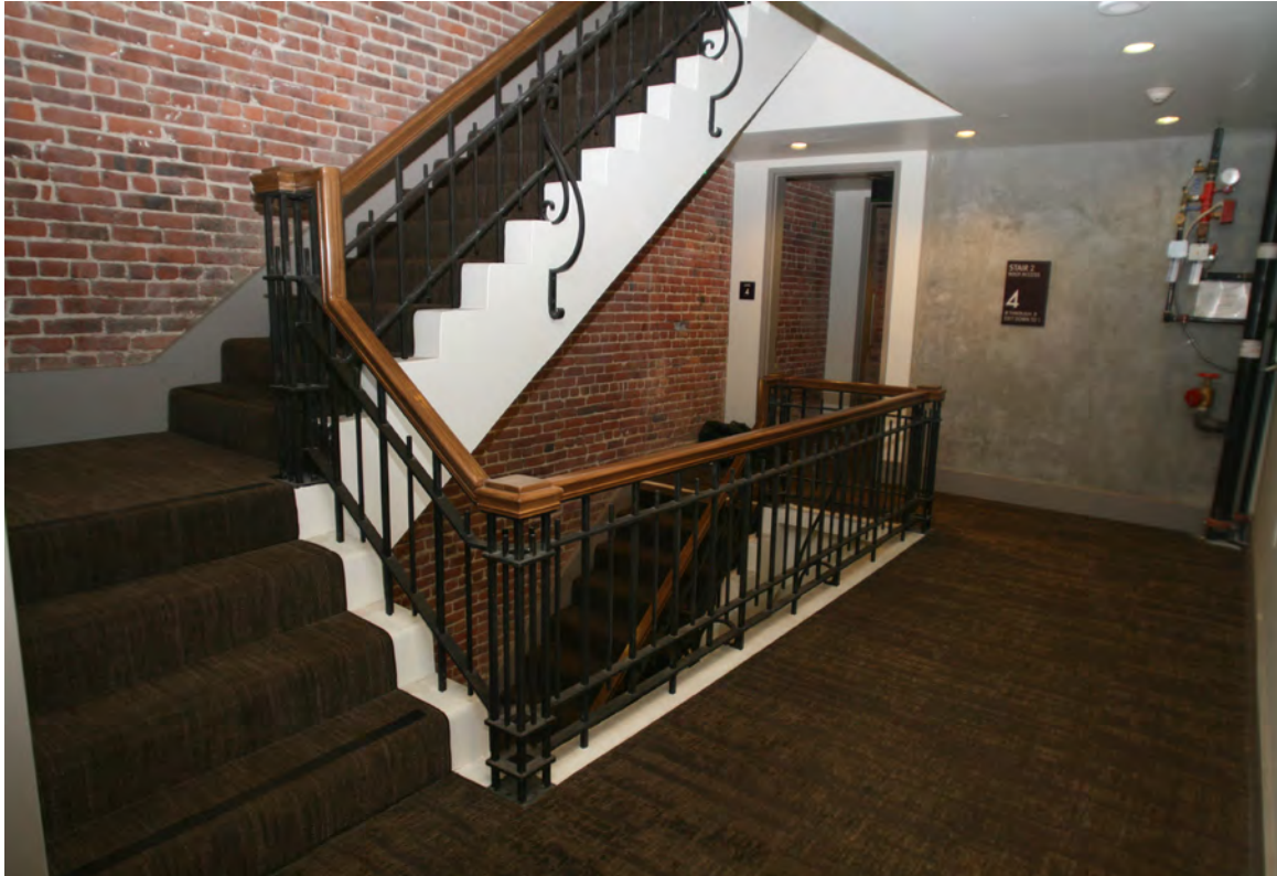
28. April 2017, Interior View, Fourth Floor, Stair at Center-East, Looking SE, Typical
