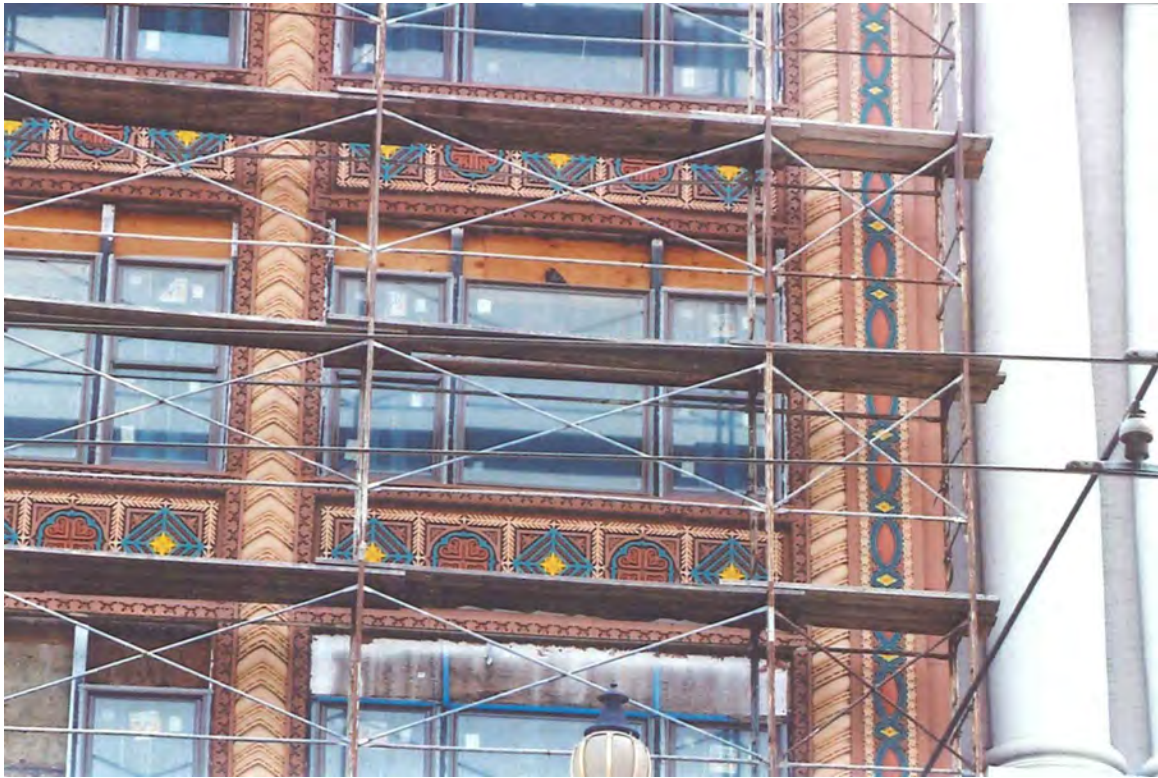
9. April 2012, Exterior Detail, North Elevation, Third Floor, Window at West, Looking S
