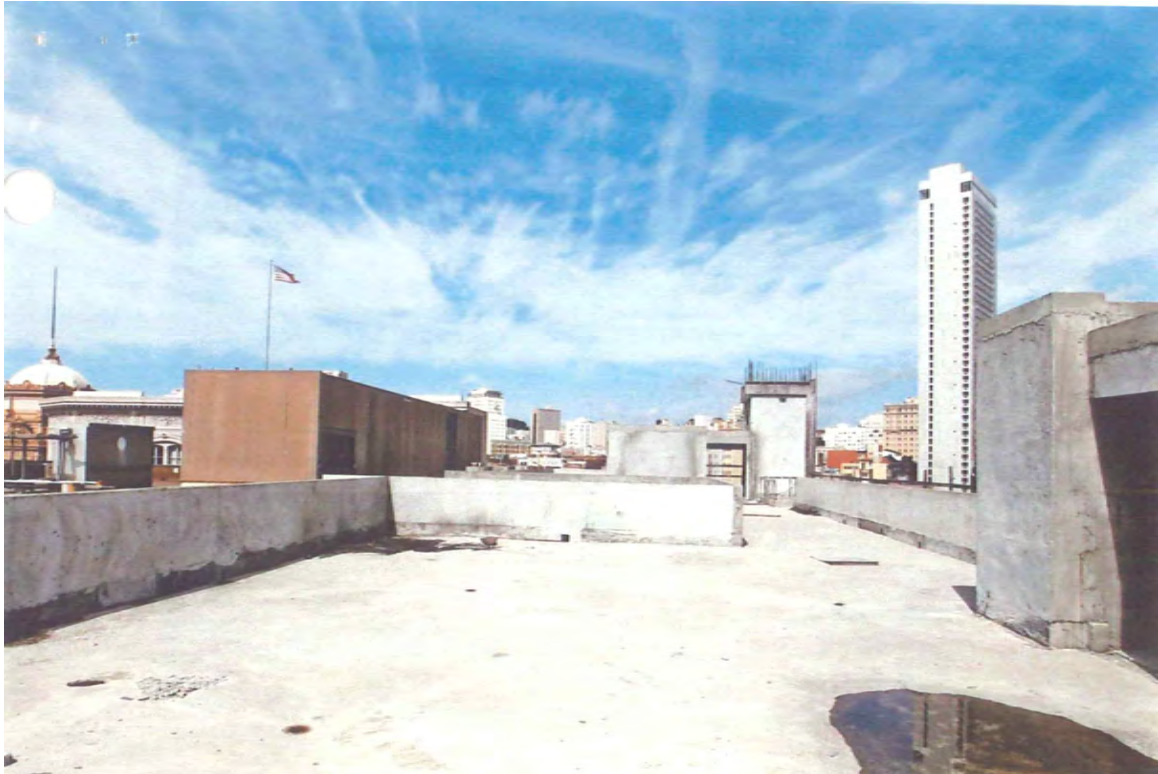
29. April 2012, Exterior View, Roof at South, Looking N
