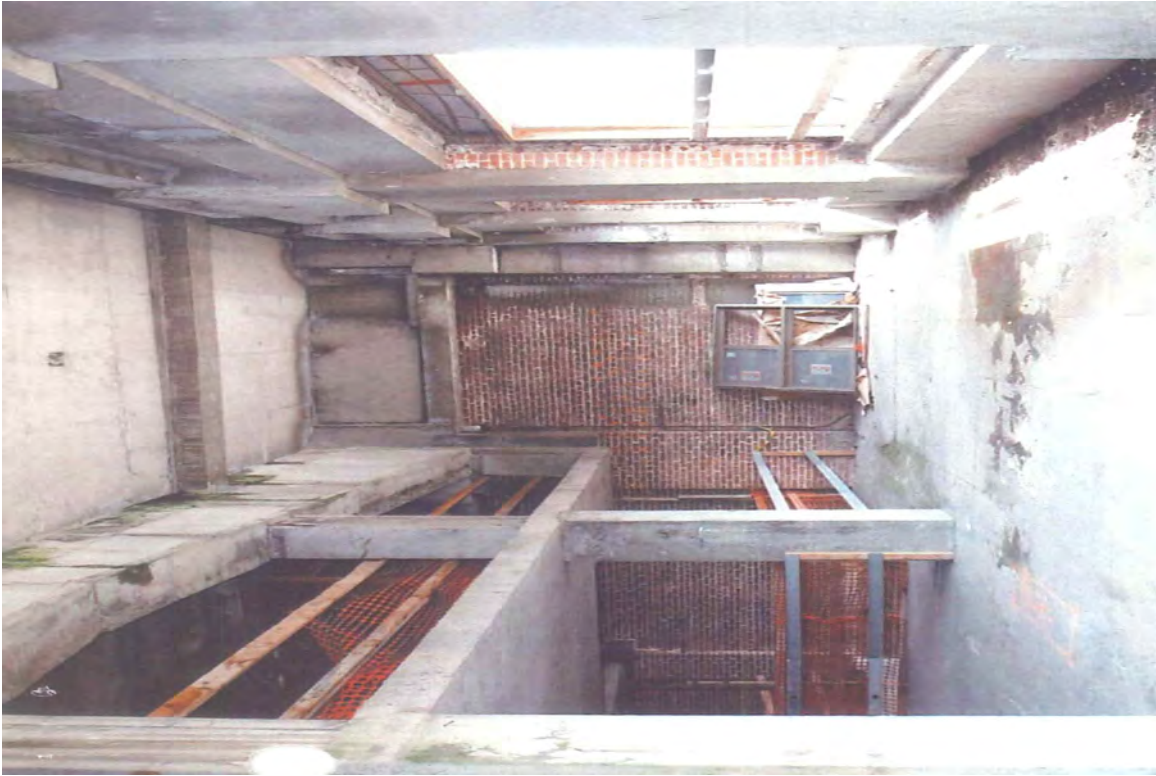
25. April 2012, Interior View, Eighth Floor at North, Looking W
