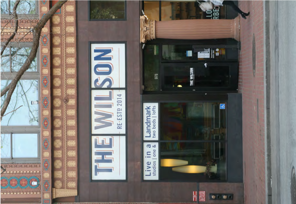
4. April 2017, Exterior Detail, North Elevation, Storefront at East, Looking S
