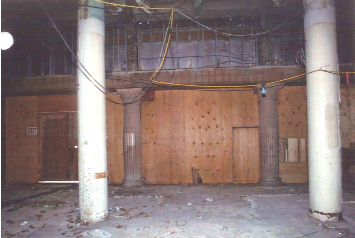
21. April 2012, Interior View, Ground Floor at North, Looking N
