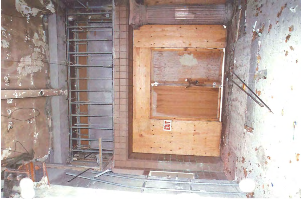
17. April 2012, Interior View, Ground Floor at Northwest, Looking N
