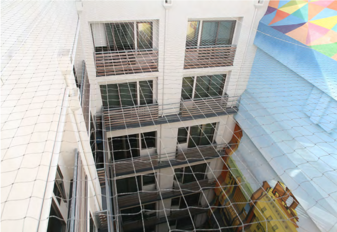
32. April 2017, Lightwell at Center-West, Looking SW
