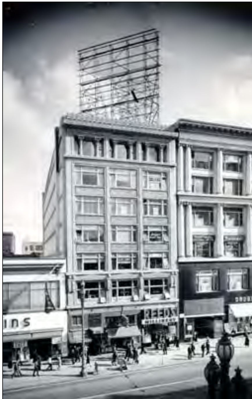
Wilson Building, May, 1944
