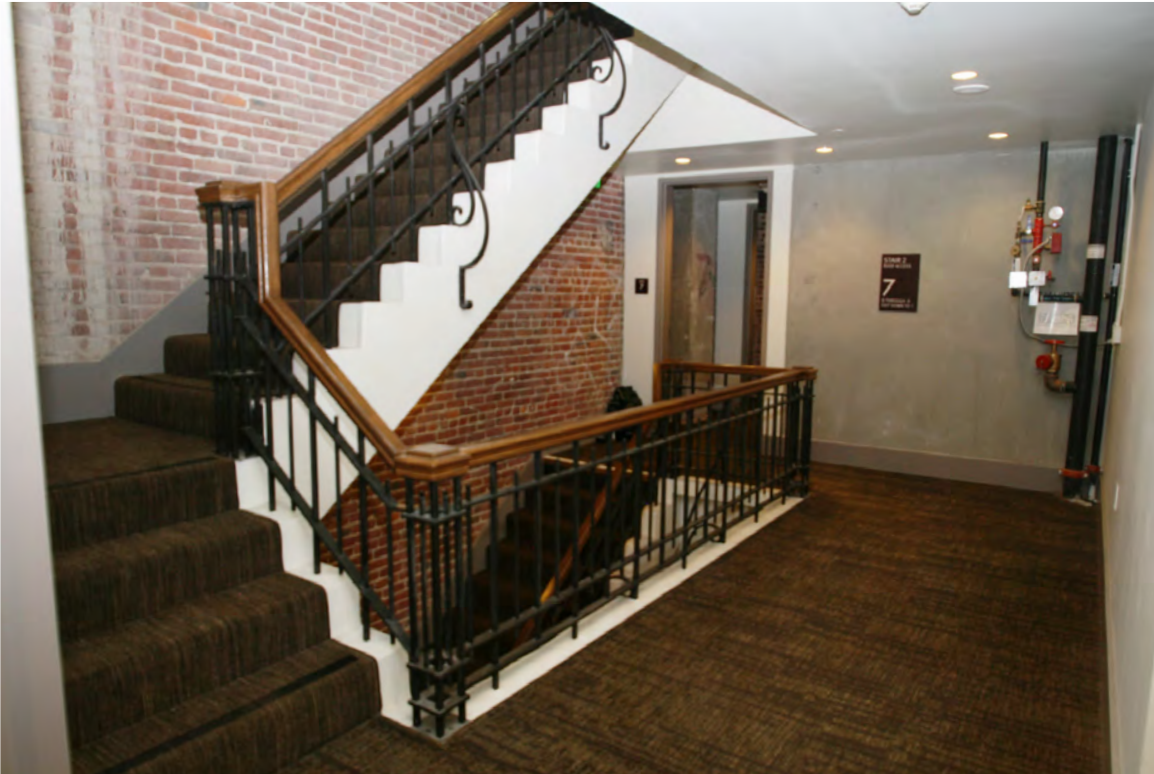
37. April 2017, Additional Photographs, Stair Landing
