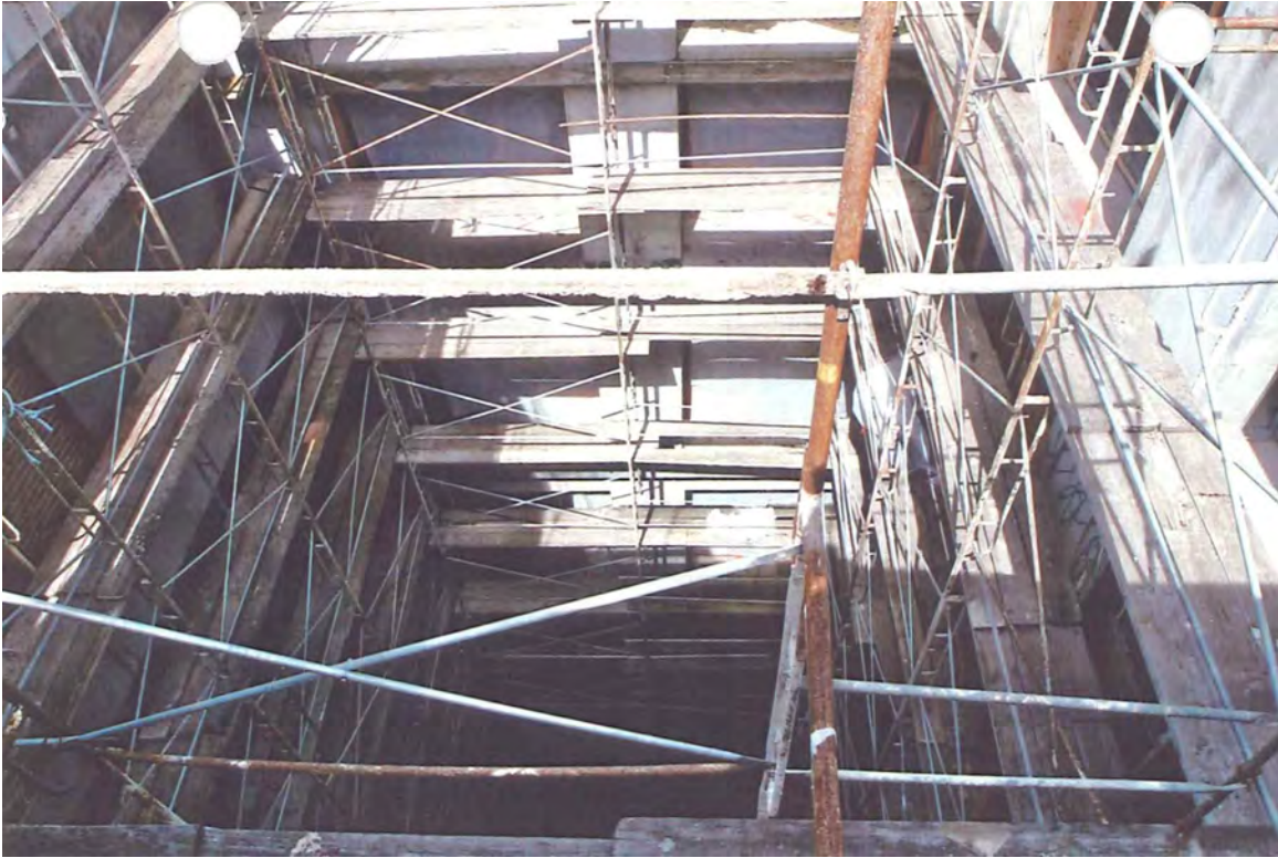
31. April 2012, Lightwell at Center-West, Looking W
