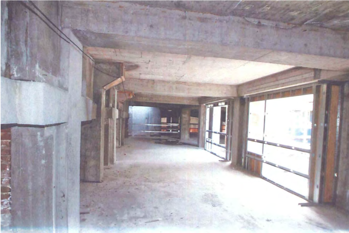
23. April 2014, Interior View, Eighth Floor at Lightwell, Looking SW, Typical
