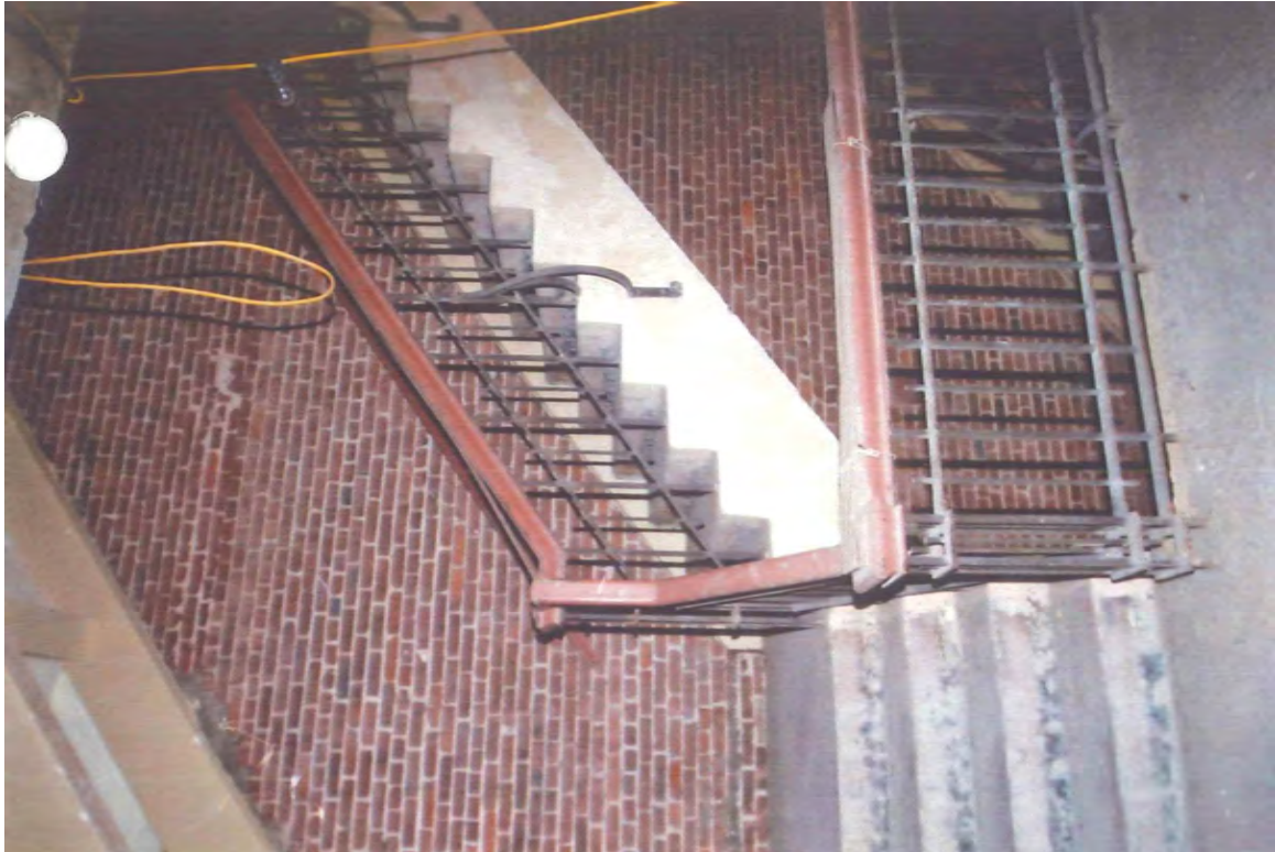
27. April 2012, Interior View, Fourth Floor, Stair at Center-East, Looking E, Typical
