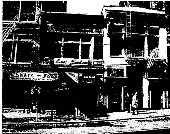
The purpose of this document is to avoid overwhelming and confusing streetscapes as shown above. In this example the signs and awnings do not correspond well to the appropriate business, extend over bays and storefronts, and they obscure the architectural features of the buildings.
