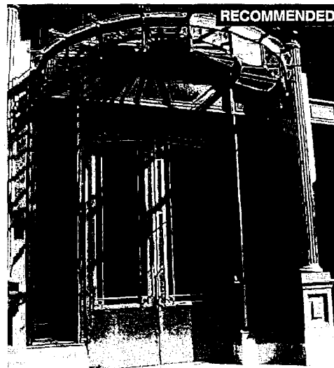
This historic storefront entrance includes a traditional door made primarily of glass and framed in bronze.
