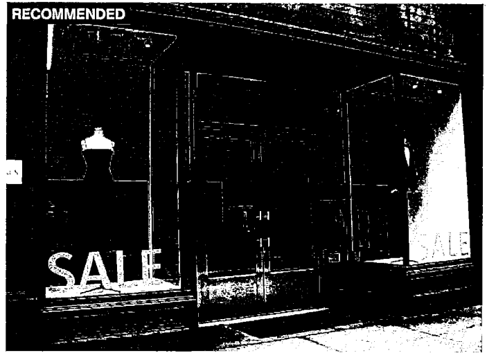
This storefront retains historic elements such as the transoms, bulkheads and piers.
