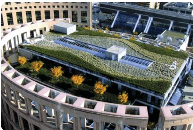
Vancouver green roof
