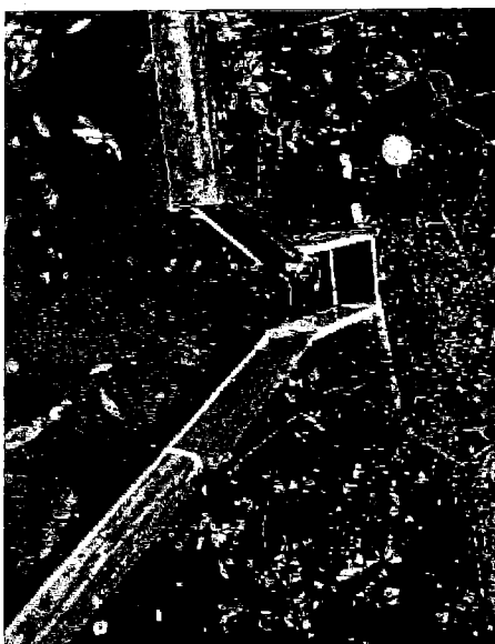
A temporary diversion structure was built upstream from a steep slope. It prevents runoff from flowing down the slope and causing hillside erosion.
