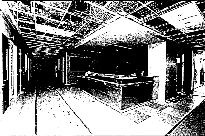
L2 - Looking Southwest at Pediatrics
