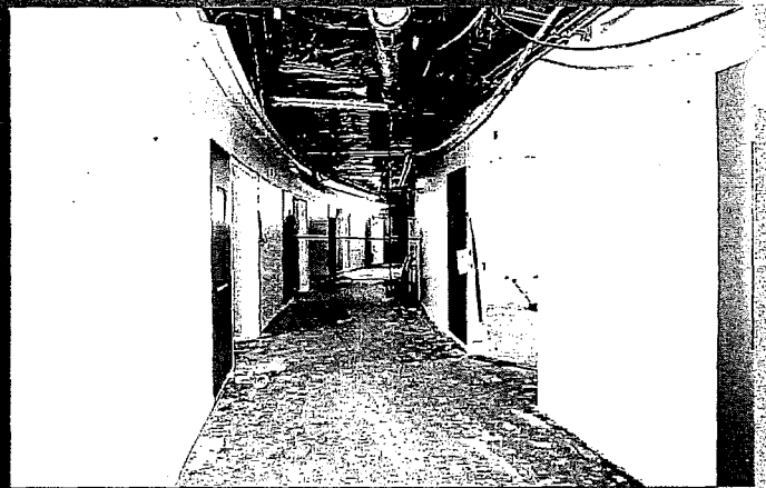
L7 - Corridor Drywall & Painting
