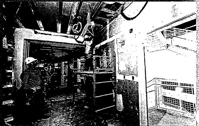
L6 - East Wall Opposite Stair 2 Landing
