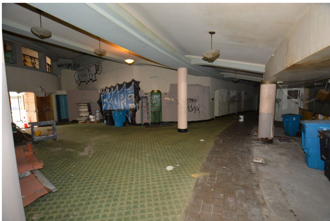
Lobby area. Note mezzanine balcony with decorative metal and wood handrail at top left. Note Art Deco pendant light fixtures with opalescent glass at top left and top center.
