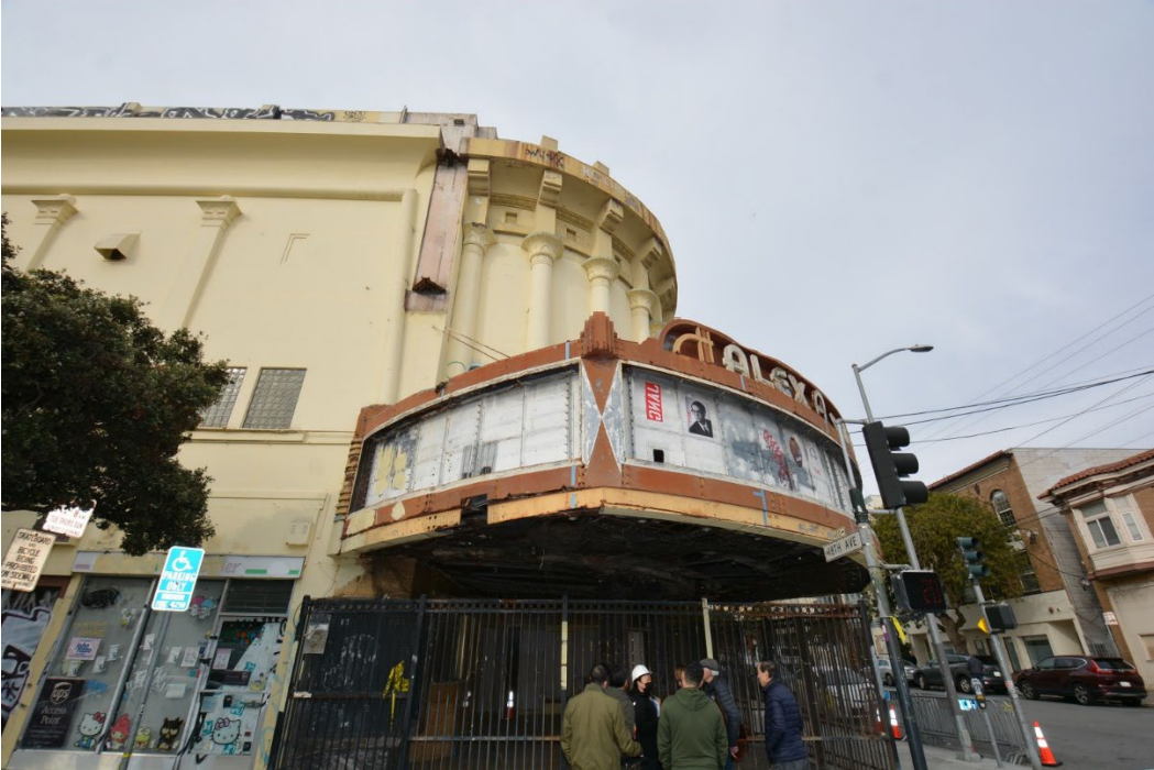
Partial view of south elevation with rectangular pilasters with squared capitals with decorative scoring, wall trims and moldings, and cornice.
