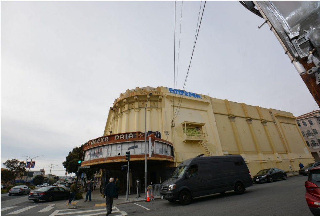
East elevation. Note rectangular pilasters with rounded shaped base and squared capitals, trims and moldings, and cornice. At corner note 1942 marquee, curved corner colonnade with rounded shaft pilasters topped with rounded capitals with papyrus leaf decorative scoring; and the entablature consisting of architrave with blind openings, foliate frieze, brackets, and a rounded cornice topped with a balustrade.
