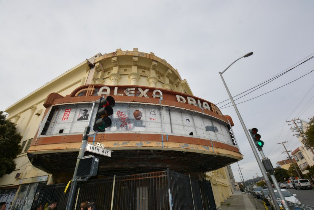
Marquee and rounded corner colonnade with pilasters with scored capitals, and brackets supporting the cornice.
