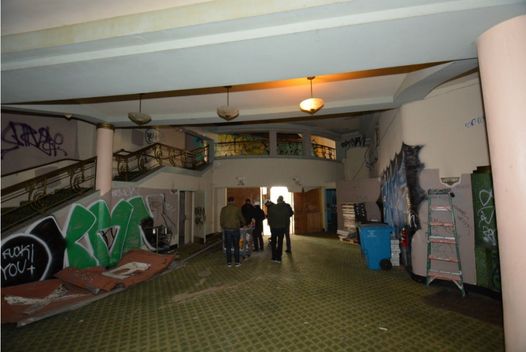
Lobby area and stairs to upper lobby balcony. Note decorative metal and wood handrail at left and Art Deco pendant light fixtures with opalescent glass at top.
