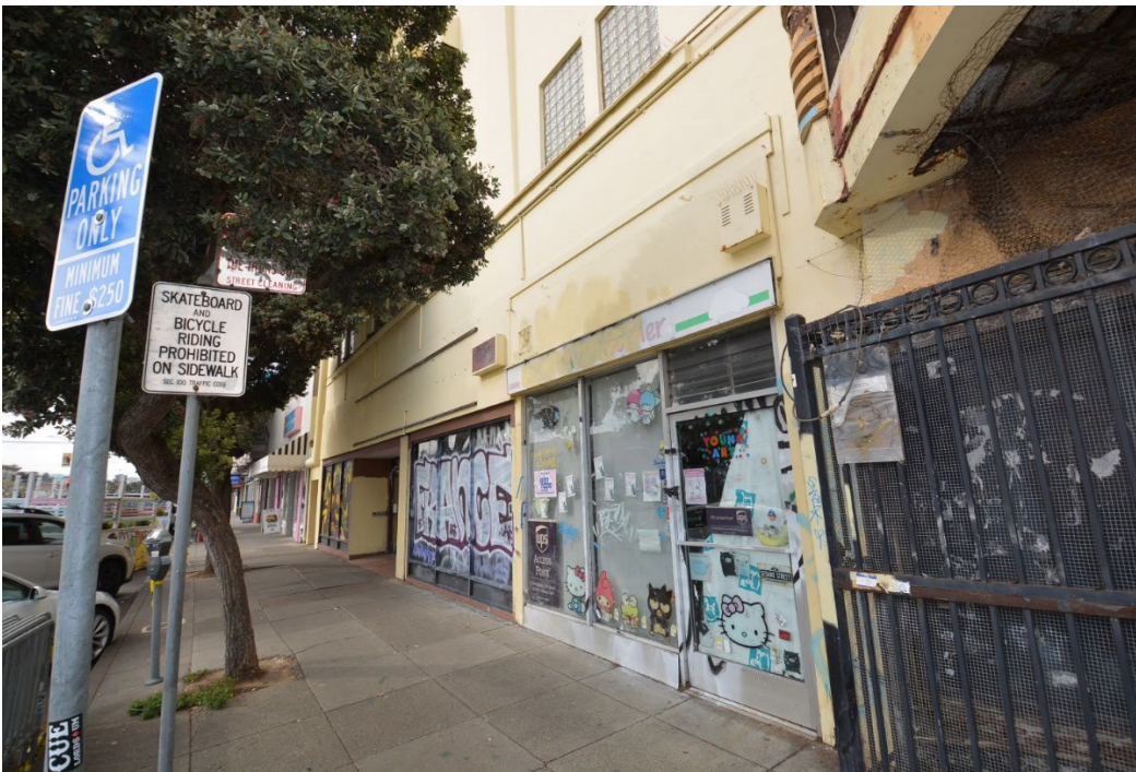
South elevation; storefronts.
