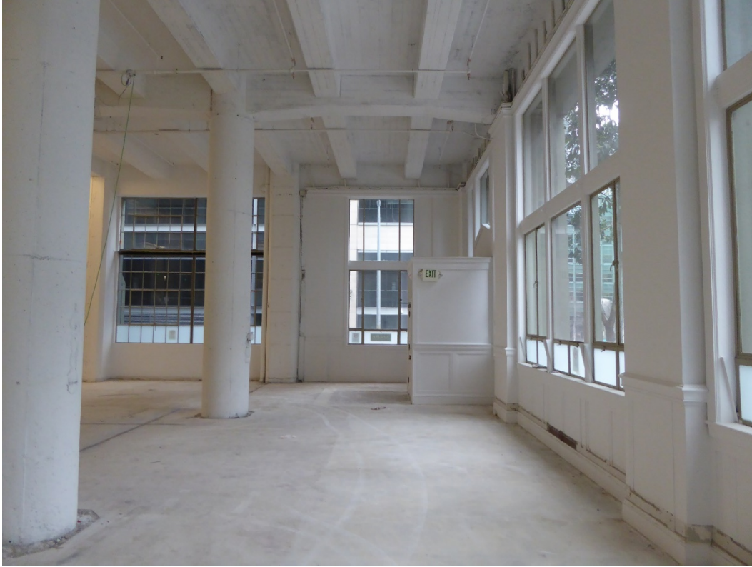
A14. View of north entry, looking northwest (ARG, February 2017).
