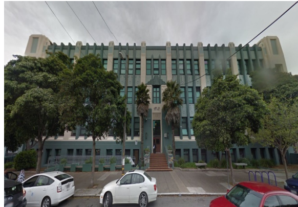
James Lick Middle School (1220 Noe Street, 1932)
