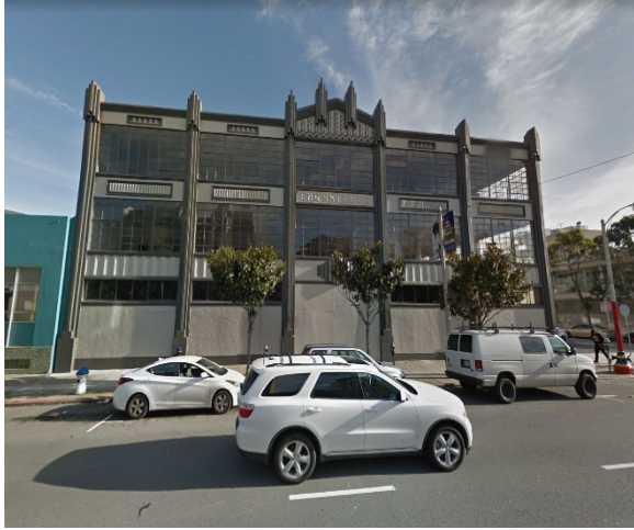
Eng-Skell Building (1035 Howard Street, 1930)
