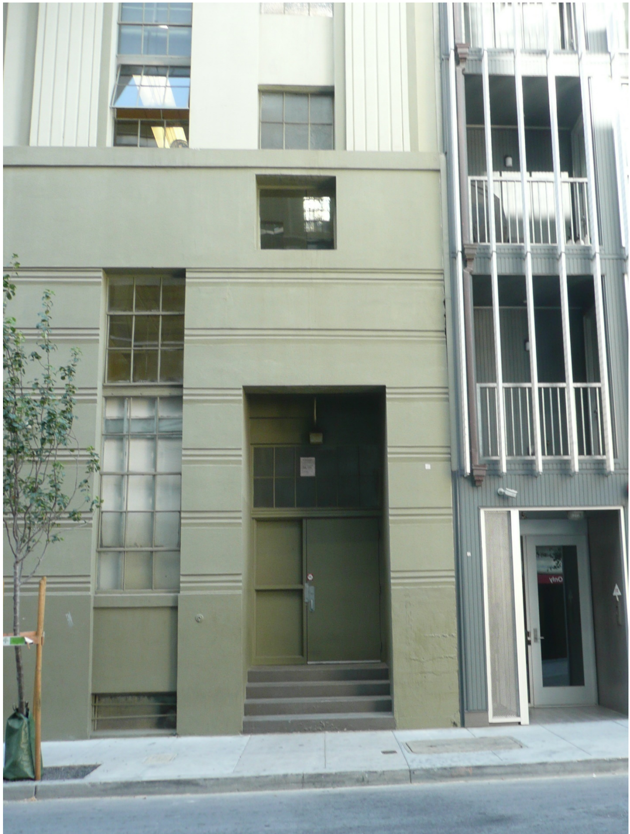
A7. Detail of entrance at west end of north façade (ARG, October 2015).
