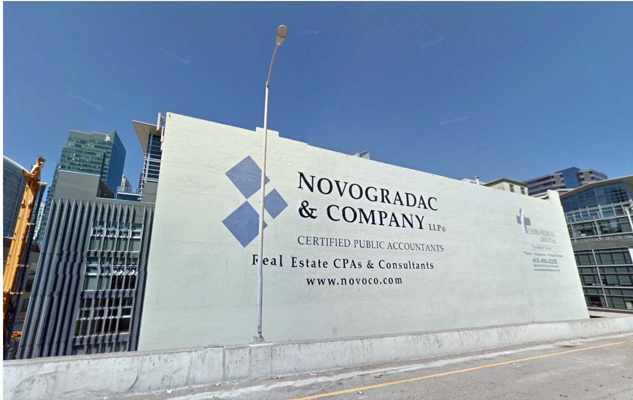
A9. View of south façade, looking north (Google street view, accessed October 2015).
