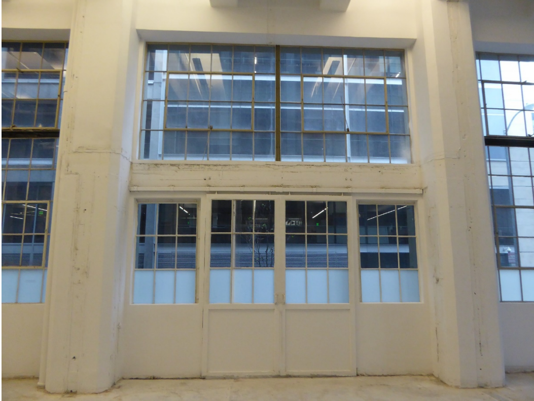
A16. View of sliding doors in the north wall of the building (ARG, February 2017). There is a matching set of sliding doors three bays to the west.
