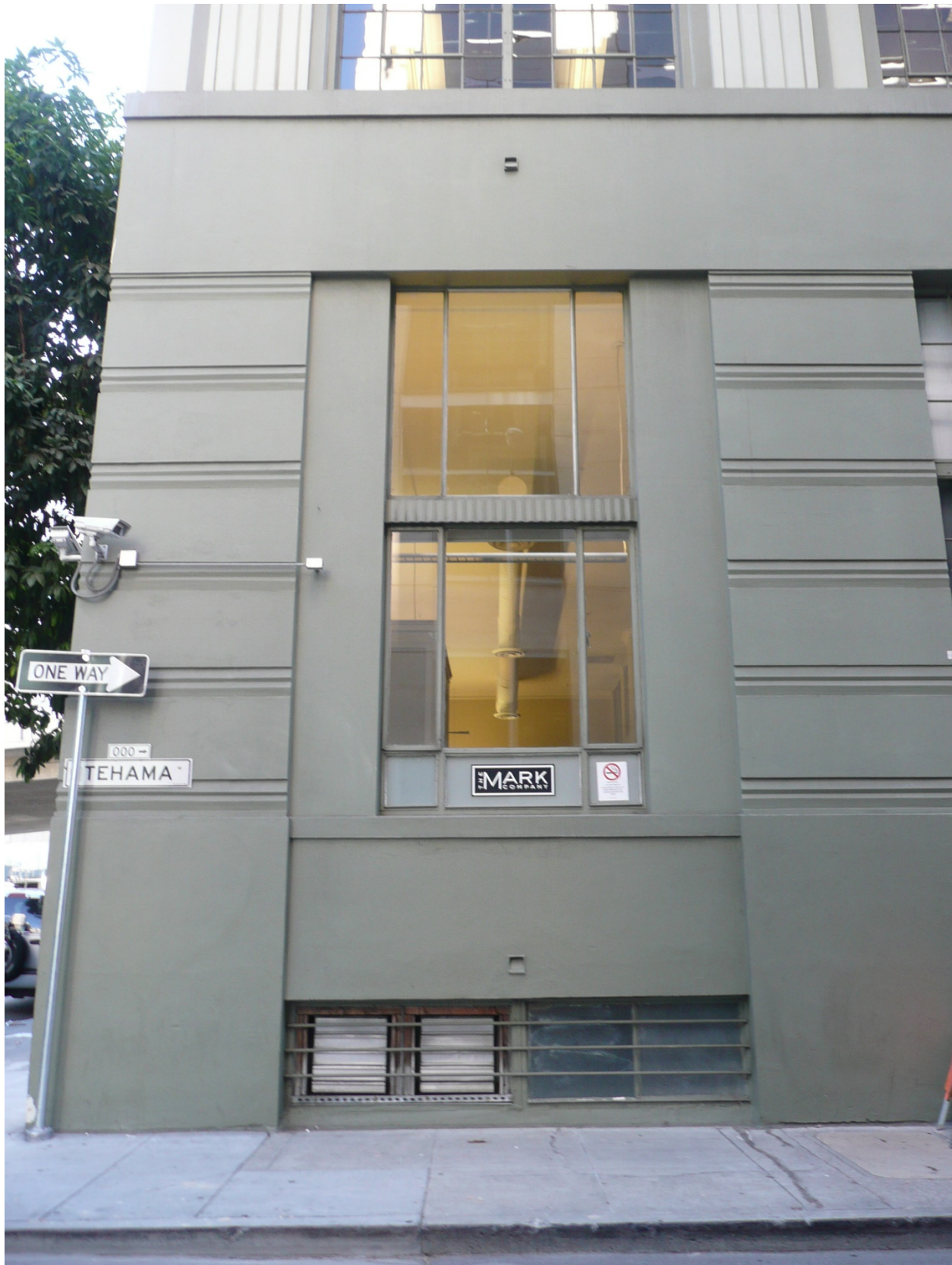
A4. Detail of easternmost bay along north façade (ARG, October 2015).
