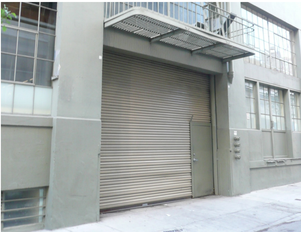
A6. View of the loading dock along the north façade, looking south (ARG, October 2015).
