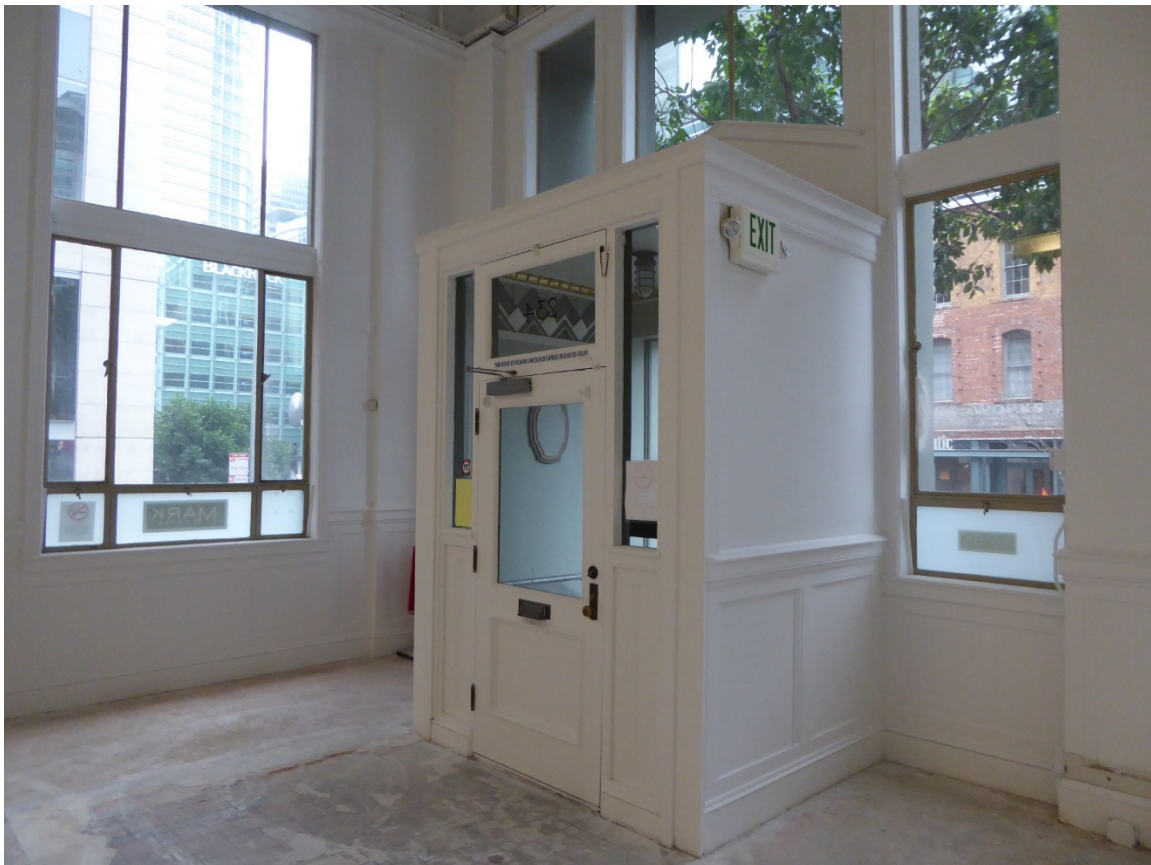
A13. Interior view of entrance at north end of front façade (ARG, February 2017). This area originally served as a display room and public space for the Phillips & Van Orden Company.
