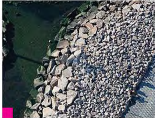
Stone edge - supplement existing edge with additional stone to create a gradient of sizes + make edge more legible
