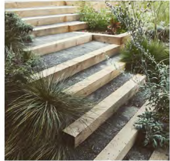
Wooden steps can be integrated into a secondary circulation system following existing topography.
