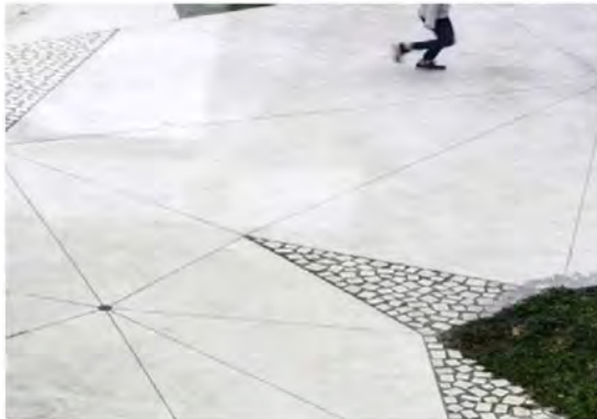
Integral color concrete with varying scales and textures add diversity to experience and relate paving back to concrete edge
