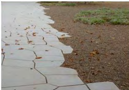
Textured/patterned concrete paving
