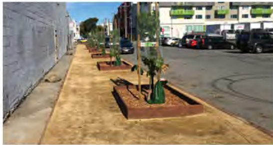
FIGURE 3-43. INTERIM PEDESTRIAN PATH ON TENNESEE STREET AT 23RD STREET
