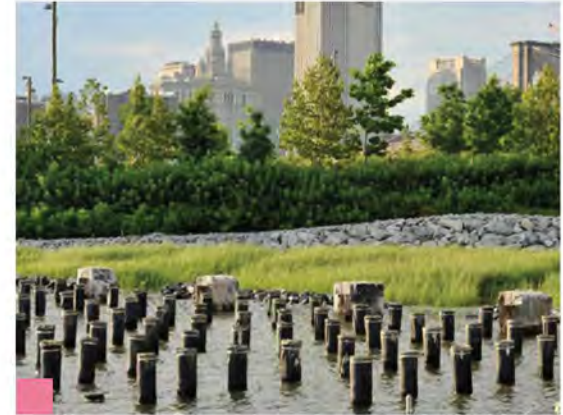
Naturalized edge - protects coast line from sea level rise while enhancing habitat value for the site
