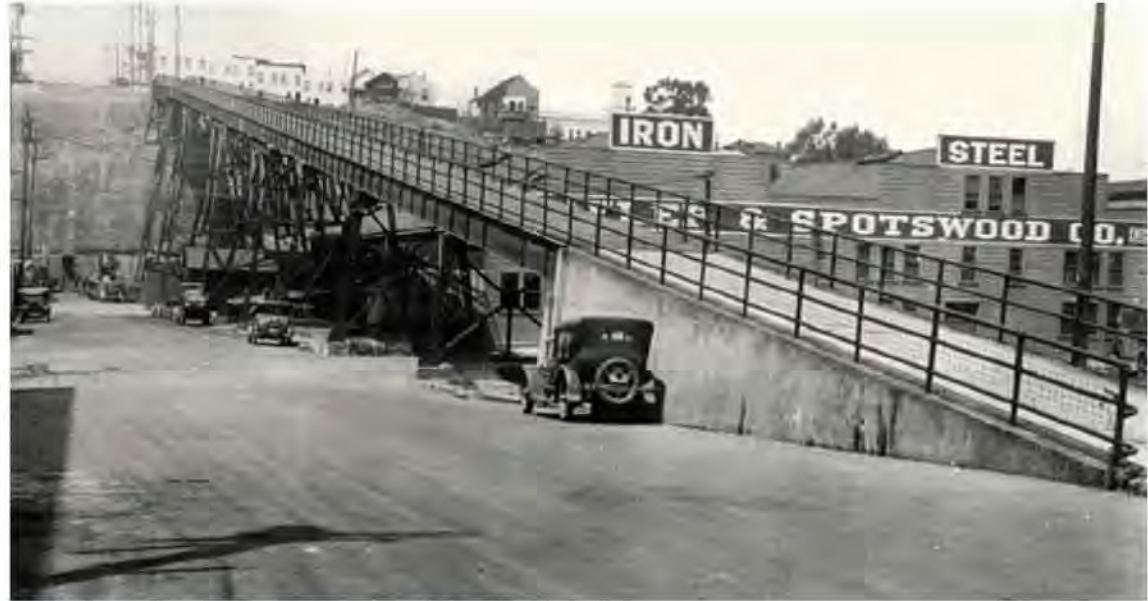
1927 19th Street viaduct as pedestrian-only bridge
