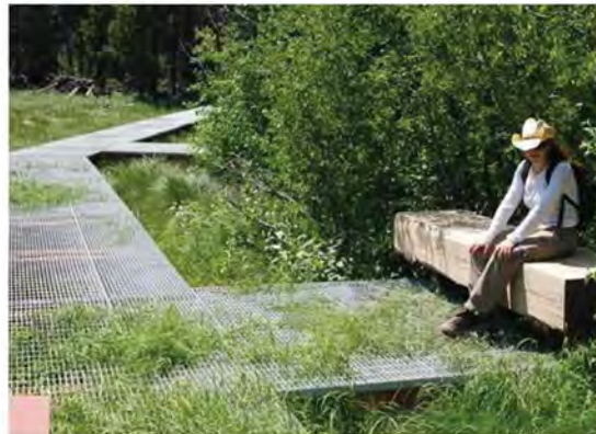
Secondary circulation - semi-transparent, raised pathways call attention to performative aspects of wetlands and help visitors feel immersed in site
