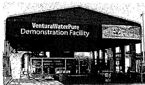
The VenturaWaterPure demonstration facility was designed to have multiple barriers for both pathogens and trace pollutants in excess of the treatment required for indirect potable reuse (IPR) via groundwater
