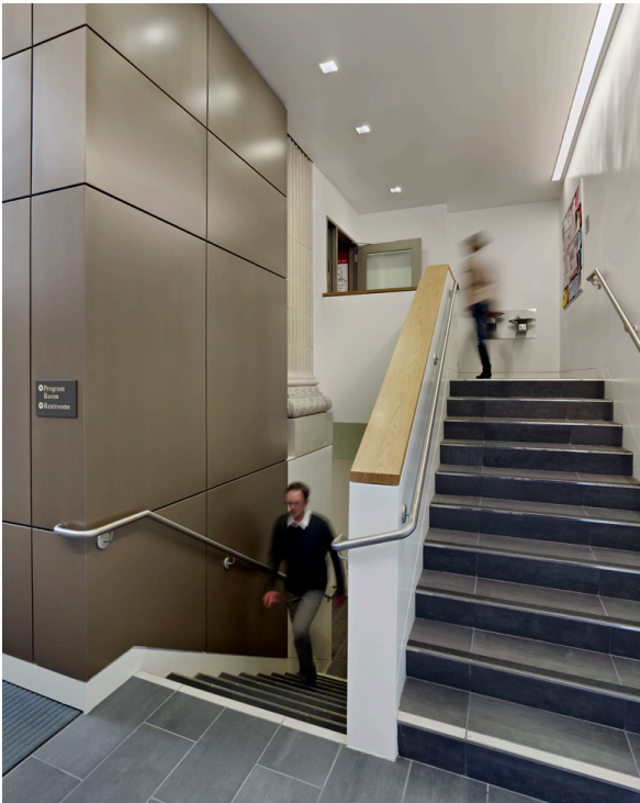
Below: Golden Gate Valley Branch Library, interior looking east at stair and elevator shaft at addition, note original exterior wall visible, 2012 after renovation. (Source: TEF Design).
