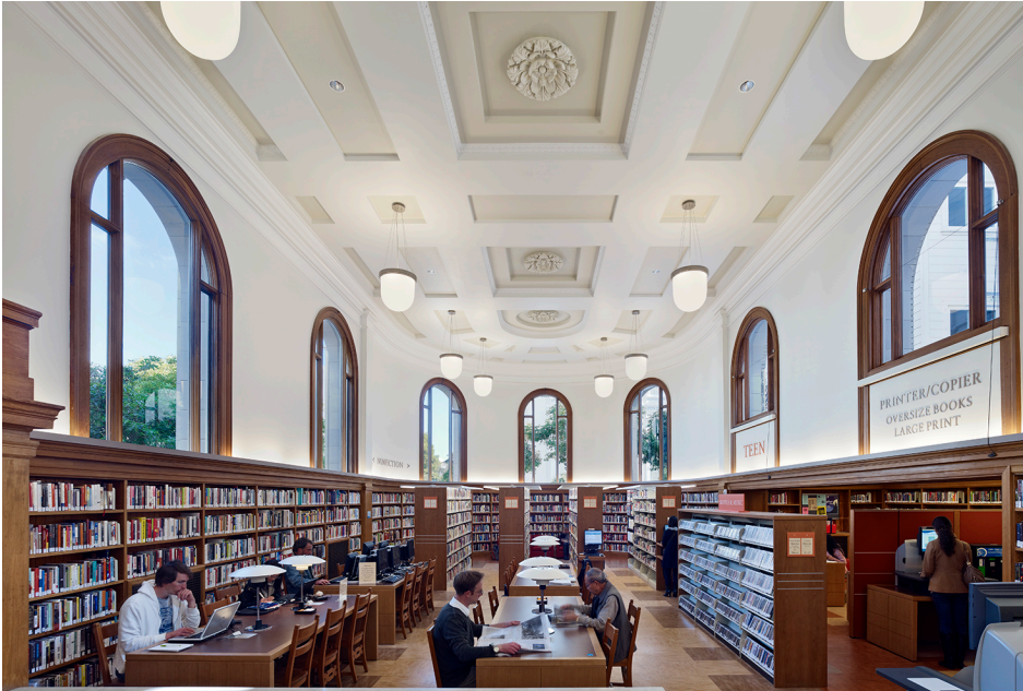
Above: Golden Gate Valley Branch Library, interior looking east, 2012 after renovation. (Source: TEF Design).
