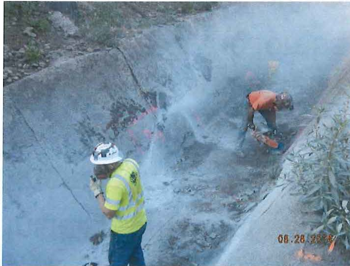
Repaired Aqueduct Lining
