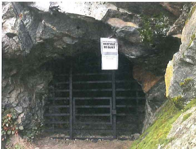
Installed Bat Gates at Adits
