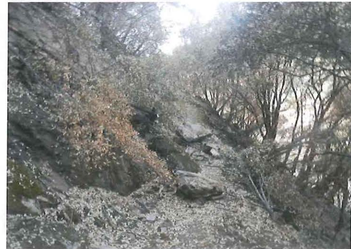
Damaged Foot Trail to Head Gates
