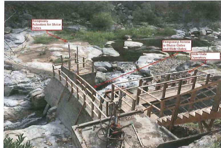
Temporary Access to Head Gates
