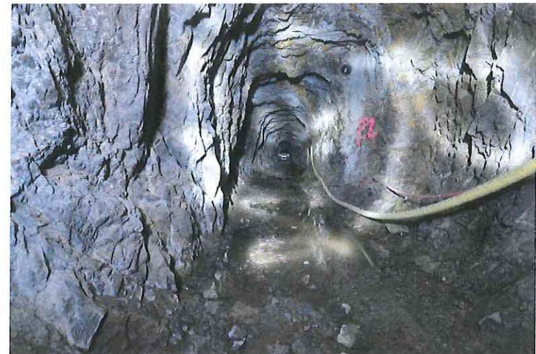
Cleaned Debris from Tunnels
