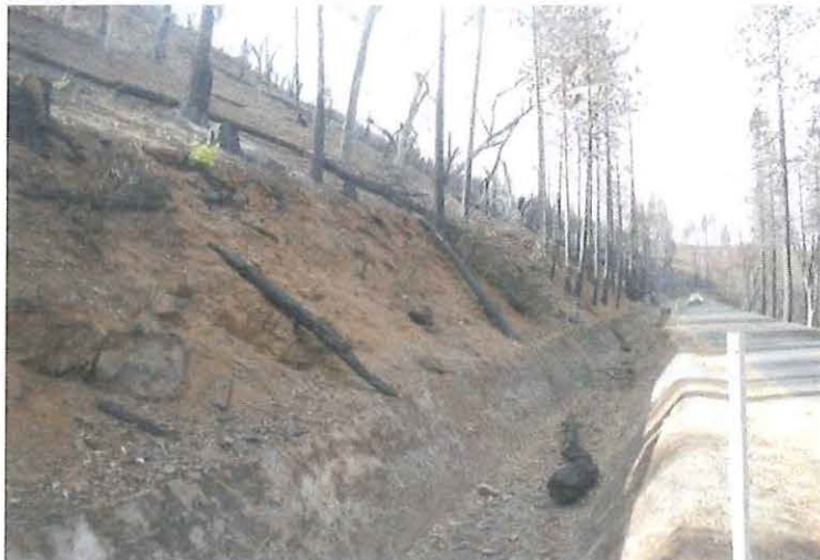
Debris from Slope
