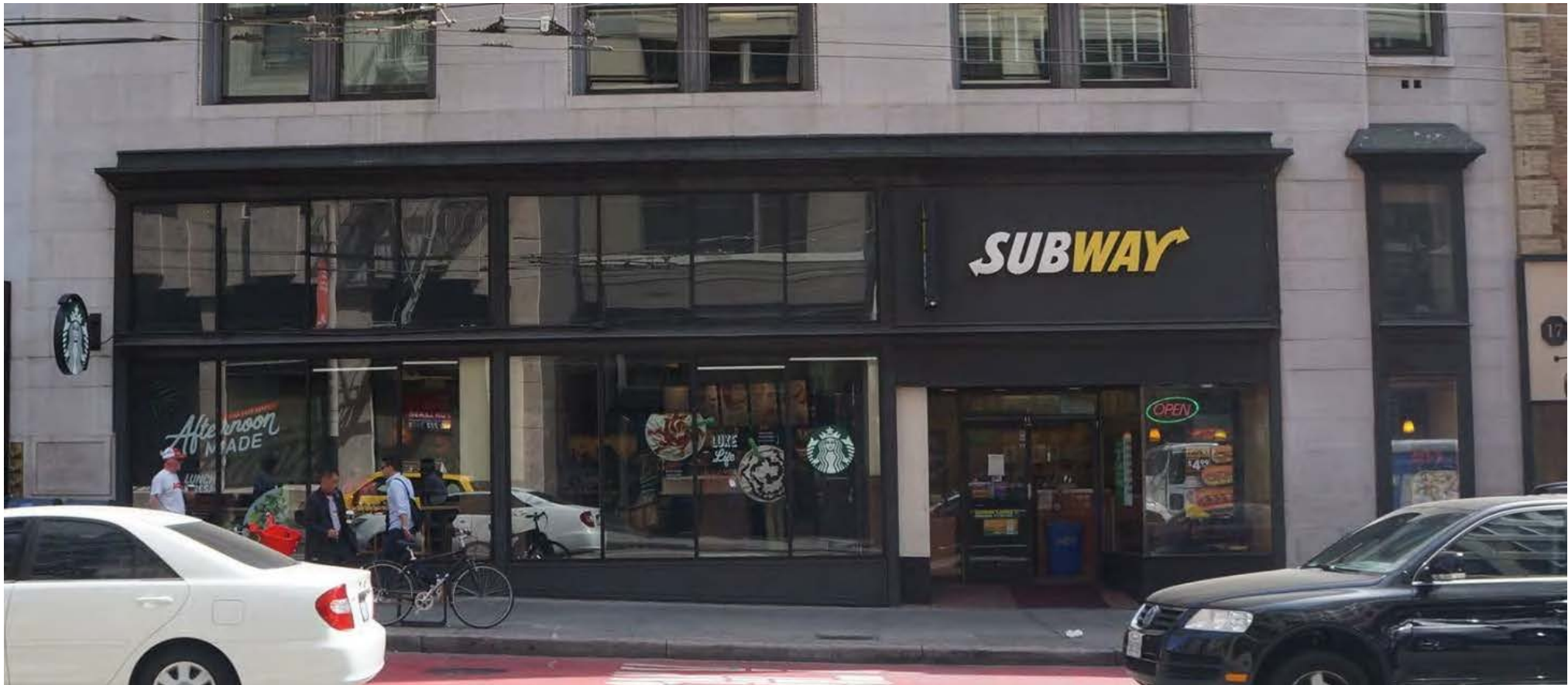
EXISTING CONDITION & REHABILITATION At the larger storefront bay at Third Street, the storefront and entryway will be replaced with a new storefront system with new sections of aluminum panels at the bulkhead where it is missing. The smaller storefront bay to the south will be reglazed and a new aluminum bulkhead will replace the existing
