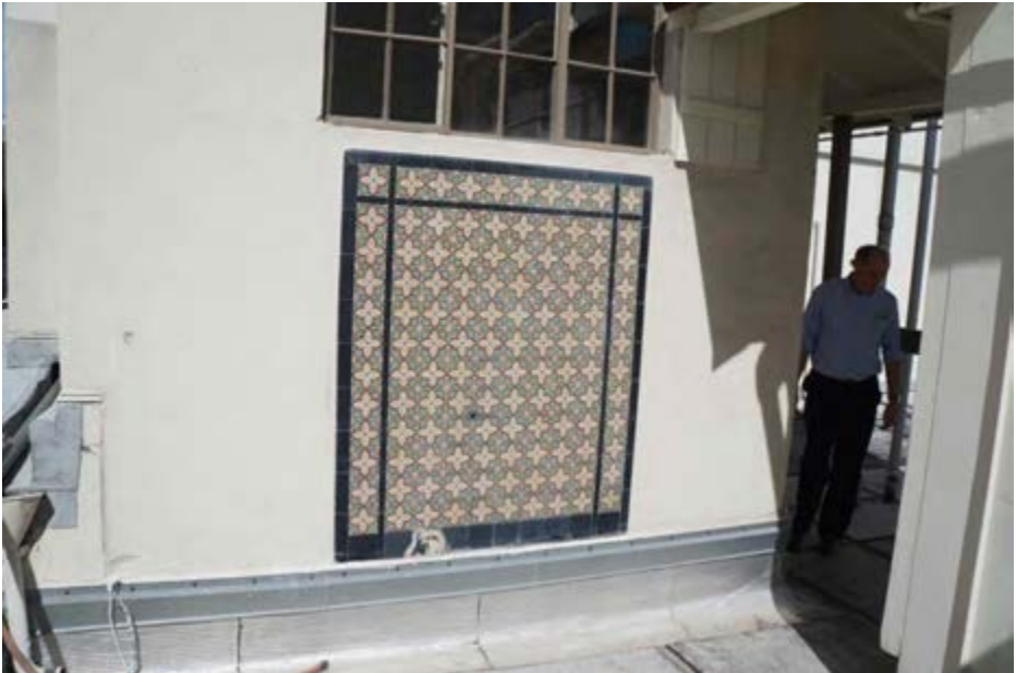
The penthouse west façade tile panel below steel sash windows.
