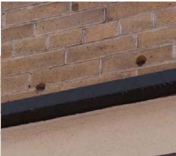
17-29 Third Street - Holes at brick and non-historic cement plaster signage where original sheet metal cornice is missing
