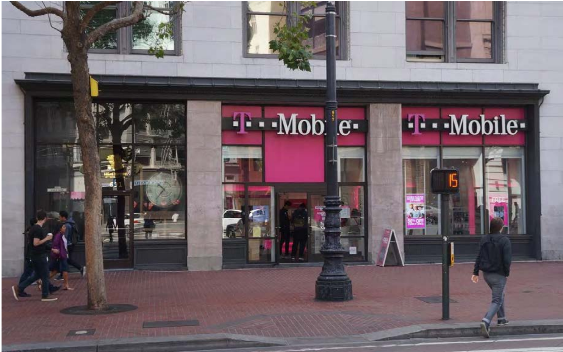
EXISTING CONDITION & REHABILITATION At Market Street, the original cast iron surround and remaining portion of the bulkhead will be cleaned and repaired. The existing aluminum storefront system will be replaced with a new aluminum storefront system and the bulkhead profile will be replicated at the center bay where it is missing.
