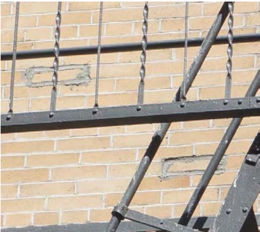
17-29 Third Street - Limited locations of mismatched mortar
