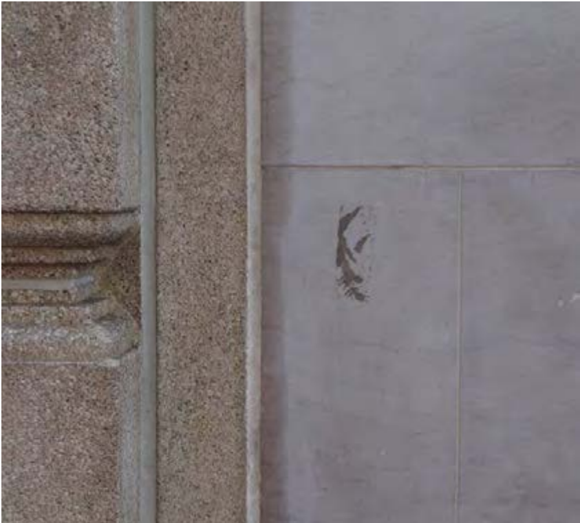
Hearst Building – Minor residue at marble podium
