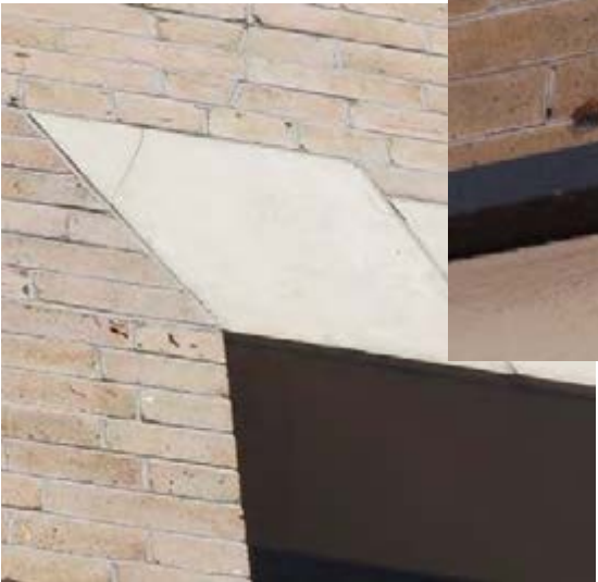
17-29 Third Street - Minor hairline crack at terra cotta
