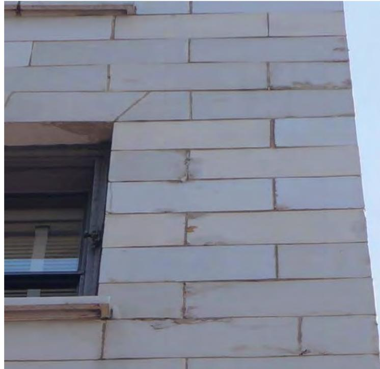
Hearst Building - Loose glazing and glaze spalls in limited
