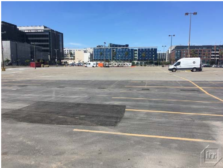
City and County of San Francisco Special Tax District No. 2020-1 (Mission Rock Facilities and Services) Terry A. Francois Blvd. San Francisco, California
