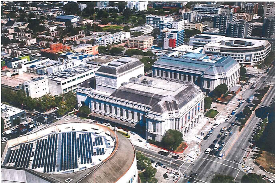
PUC solar panel installation on Davies Symphony Hall.
